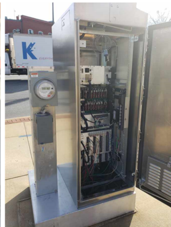
Main Street and Augusta Street / River Street
