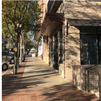
Sidewalks Crash Reduction = 65-85% Paved Shoulder Crash Reduction = 71%
