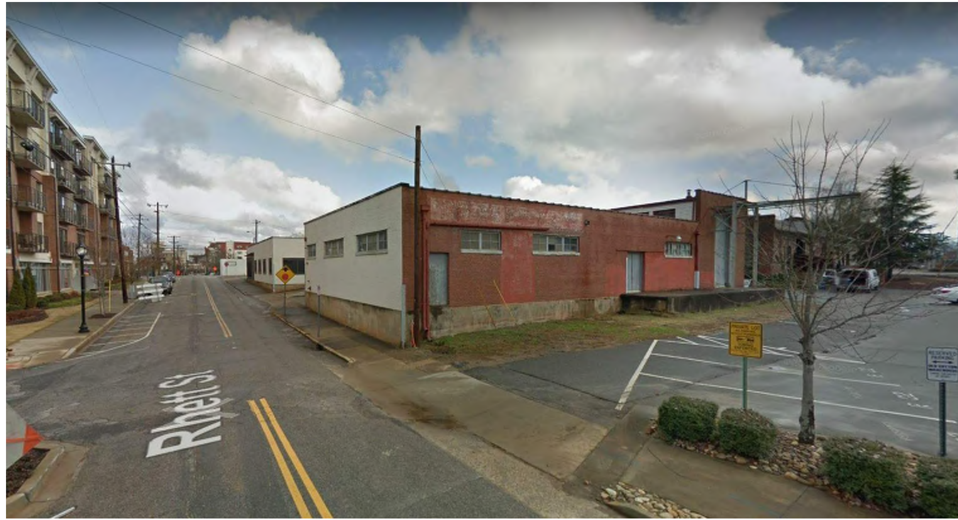
5 - VIEW OF EXISTING REAR LOADING DOCK FROM RHETT STREET
