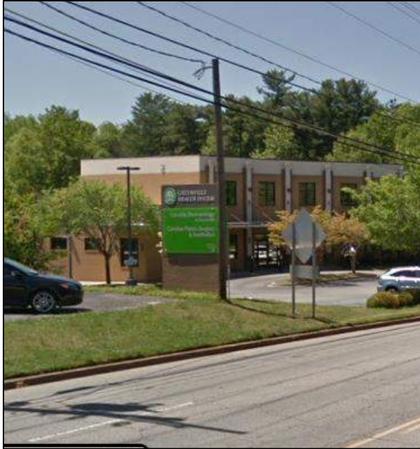
Existing Sign Face
