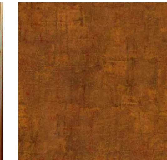
EXTERIOR CLADDING IRON CORTEN - RUST RUN-OFF MITIGATED THRU DRAINAGE DESIGN
