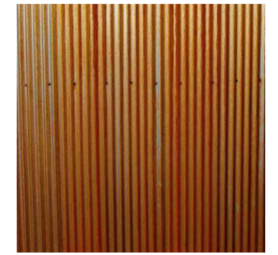
METAL ROOF AND ENTRY AWNING IRON CORTEN - RUST RUN-OFF MITIGATED THRU DRAINAGE DESIGN
