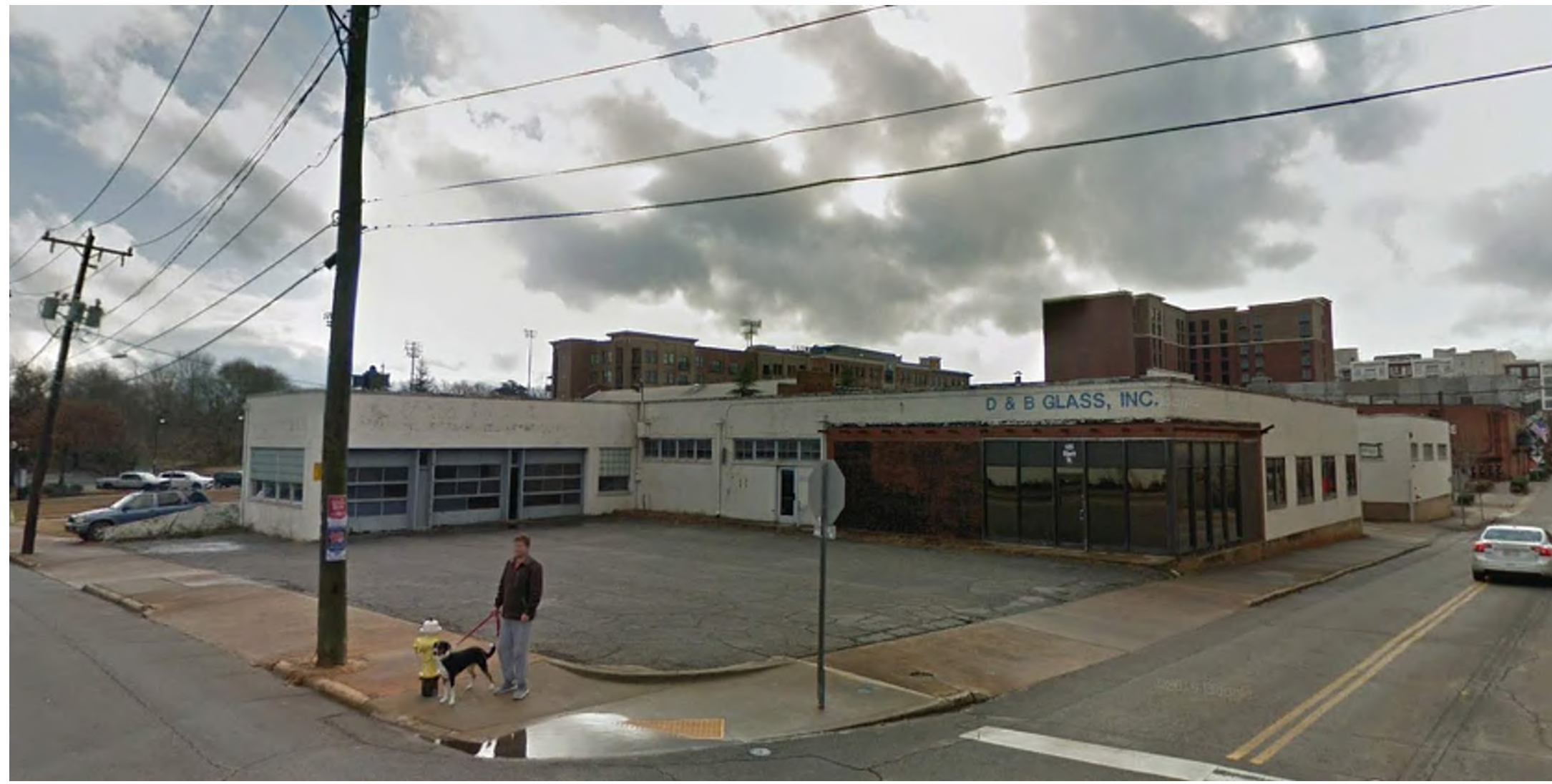
2 - STREET VIEW FROM CORNER OF WARDLAW AND RHETT STREET
