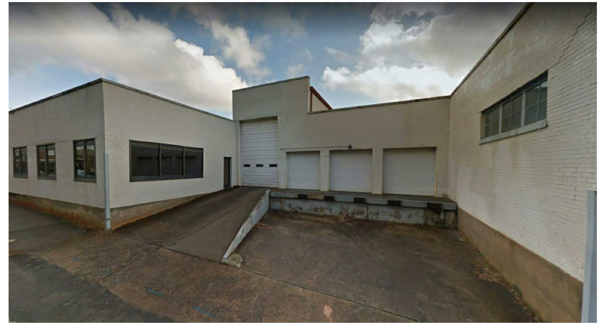
4 - VIEW OF EXISTING LOADING DOCK FROM RHETT STREET
