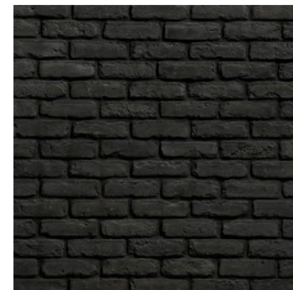
EXISTING BRICK EXISTING BRICK - TO BE PAINTED
