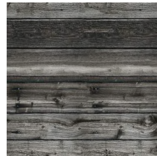
EXTERIOR CLADDING RECLAIMED BARN WOOD
