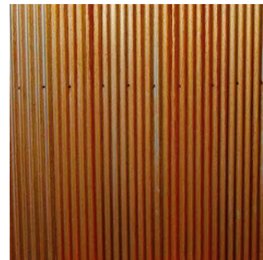
METAL ROOF AND ENTRY AWNING IRON CORTEN - RUST RUN-OFF MITIGATED THRU DRAINAGE DESIGN
