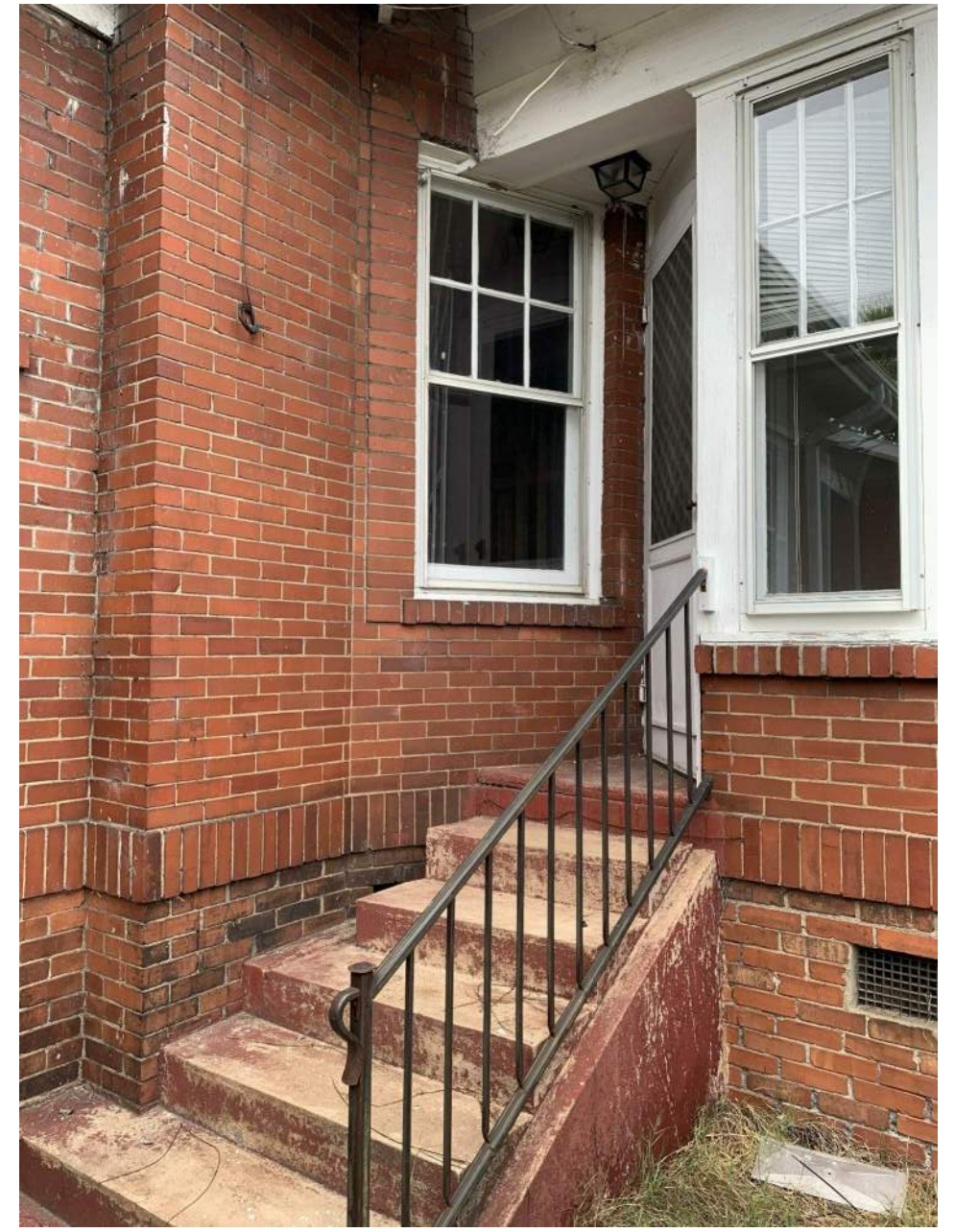
REAR STAIR AND PORCH CONNECTION
