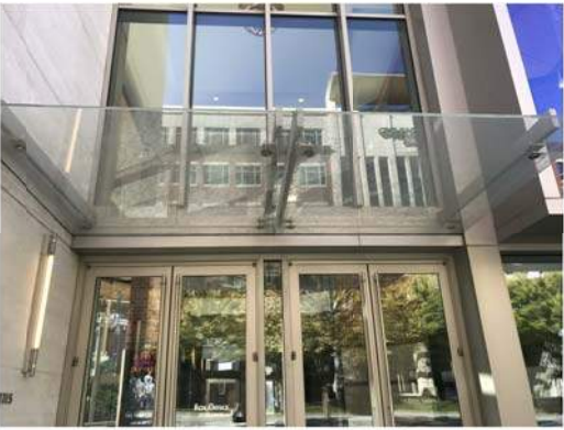
CPY-G FRITTED GLASS CANOPY (SIMILAR TO MAIN CONCERT HALL) PAINTED STEEL STRUCTURE
