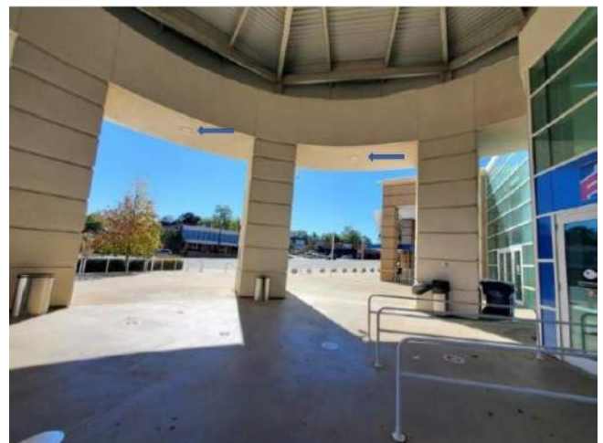
Outer Edge Lighting (5 total)
