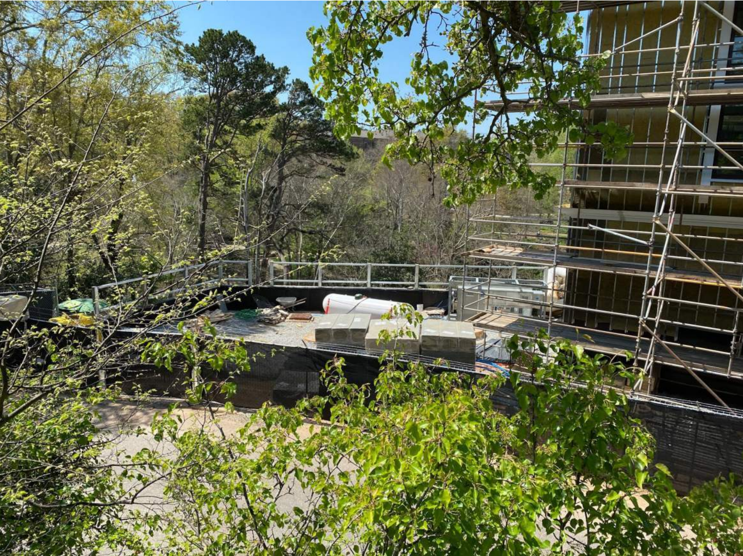
View of hotel service area on Falls St
