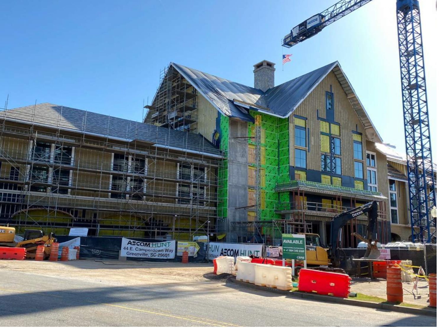
Construction progress of plaza side of Bohemian Hotel
