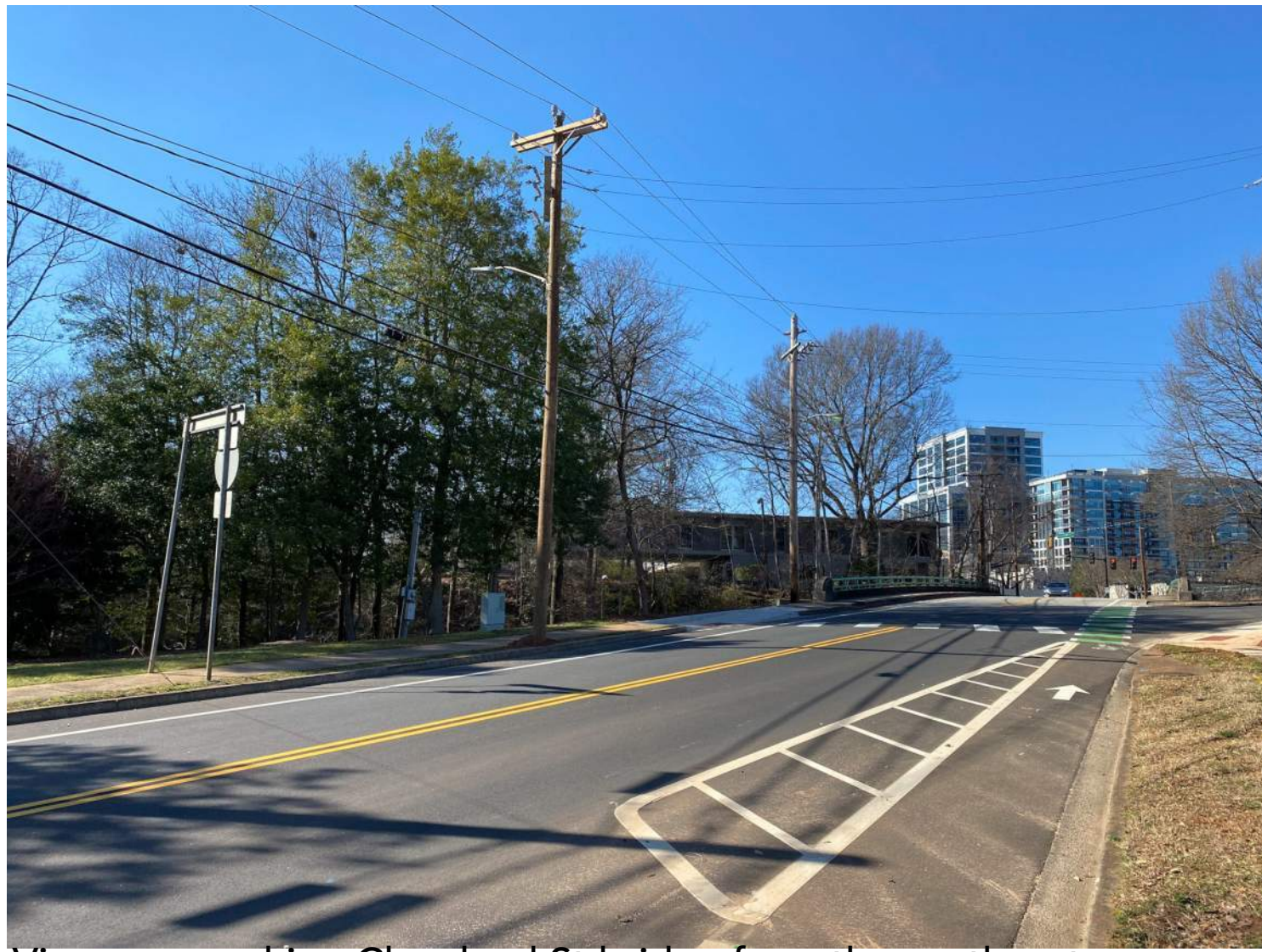
View approaching Cleveland St bridge from the southeast
