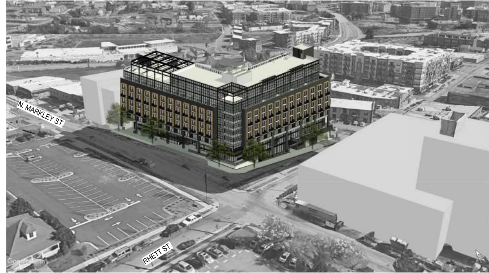
MAIN CORNER SITE VIEW LOOKING NORTH-WEST
