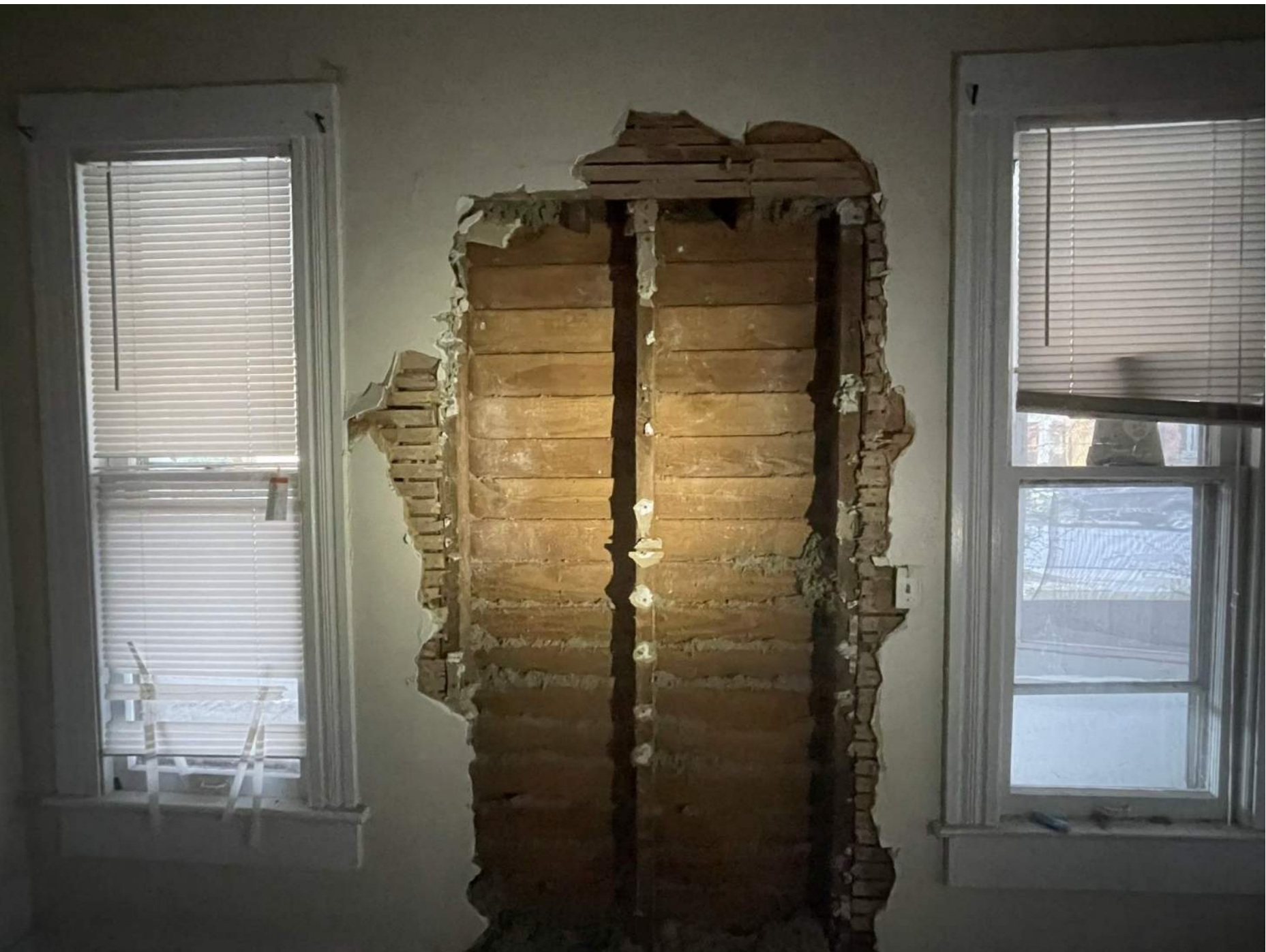
EVIDENCE OF ORIGINAL DOOR LOCATION
