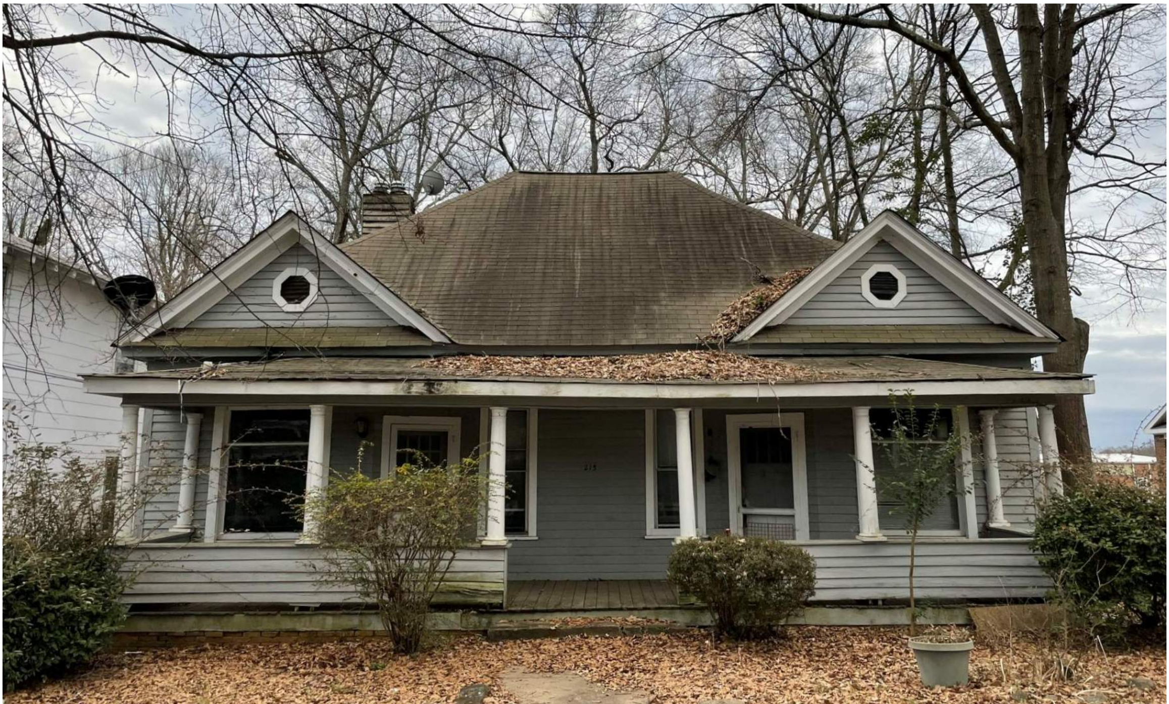
EXISTING NORTH (EARLE STREET) VIEW
