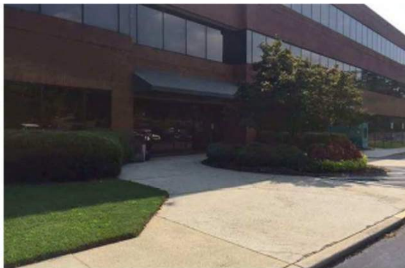
16 - View of western facade of AGFA building
