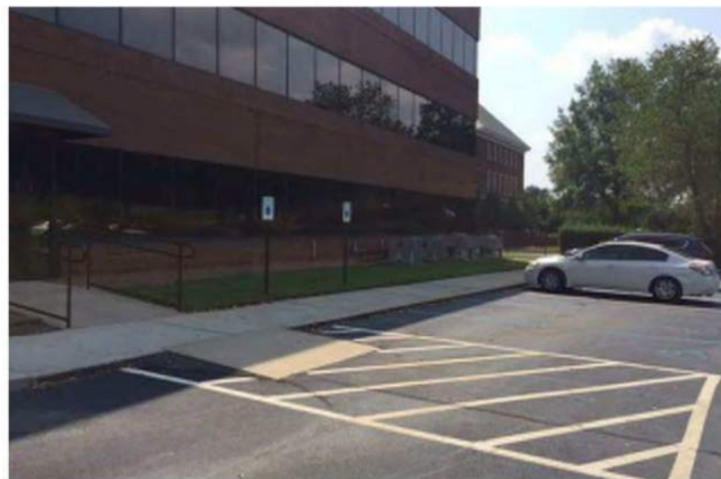
17 - View of western facade of AGFA building
