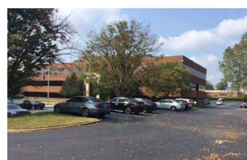
9 - View of north east corner of AGFA building
