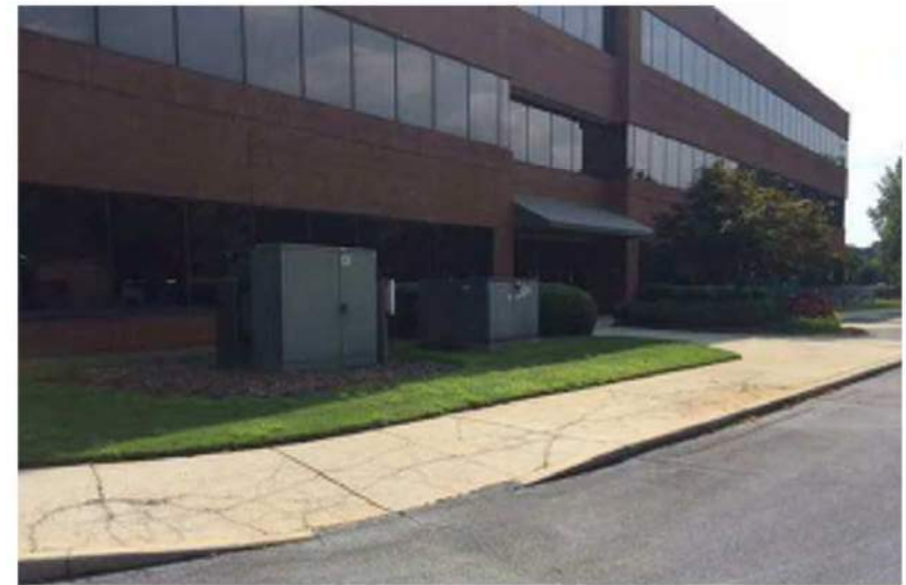
15 - View of western facade of AGFA building
