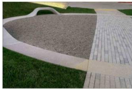
(1.4) CONCRETE BANDING FLUSH WITH PAVERS
