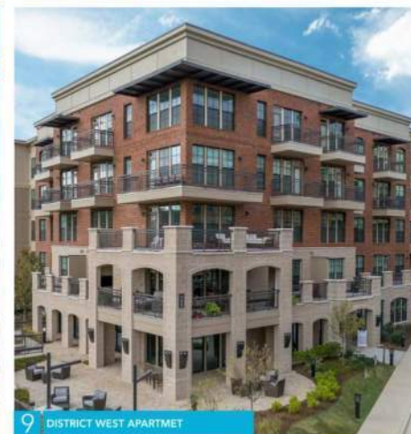
9 DISTRICT WEST APARTMET
