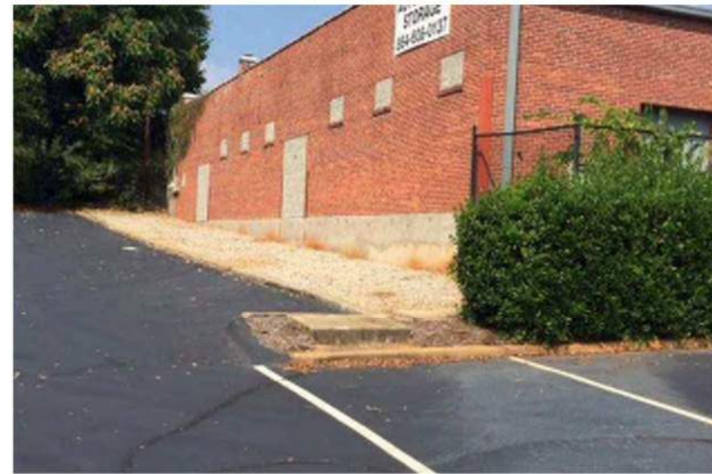
2 - Existing building along western property line.
