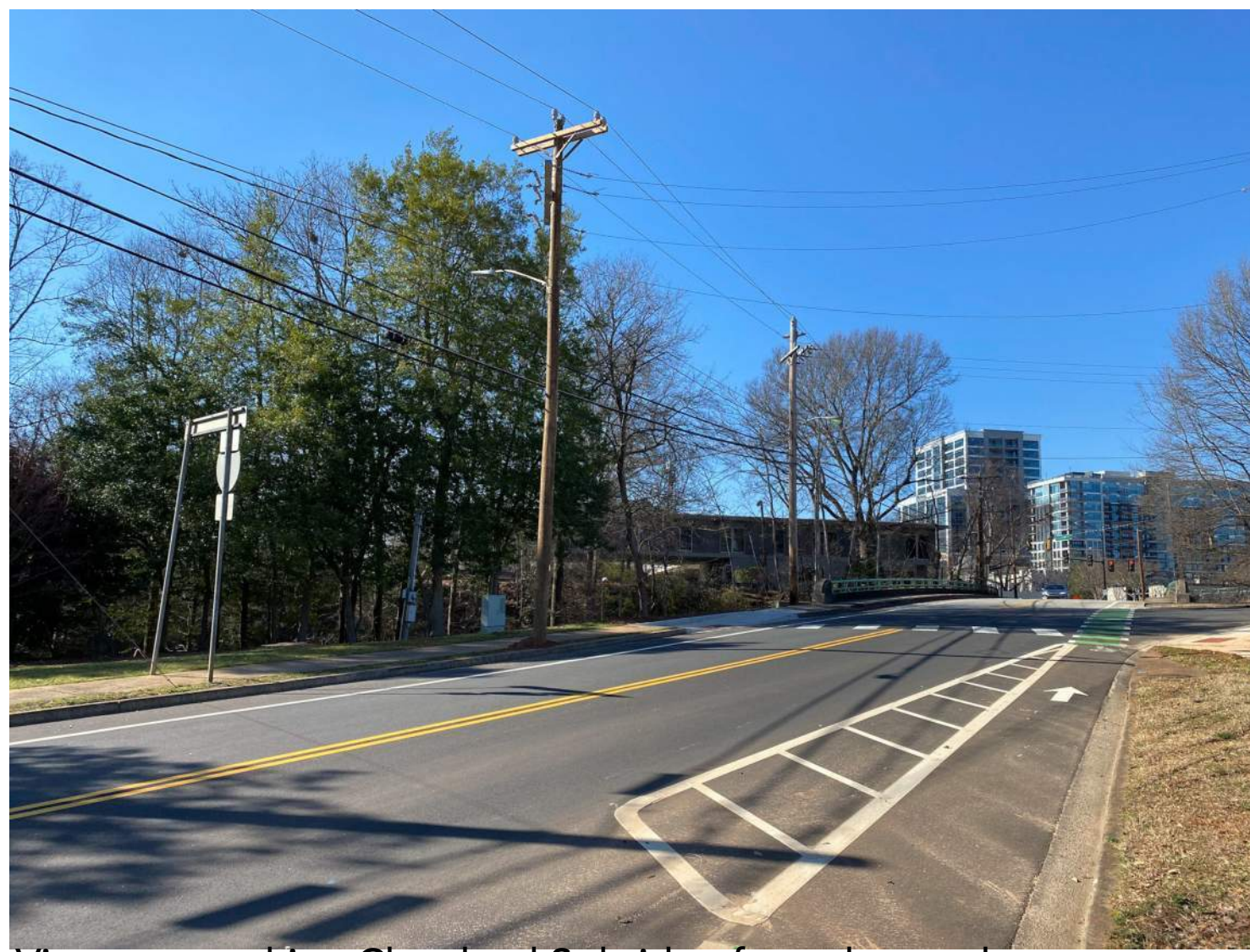
View approaching Cleveland St bridge from the southeast
