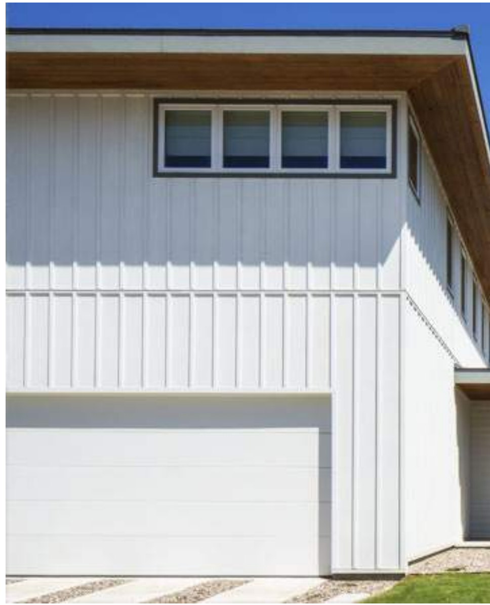
FIBER CEMENT SIDING LAP | BOARD AND BATTEN | SHIPLAP - MANUFACTURER AND FINISH T.B.D.
