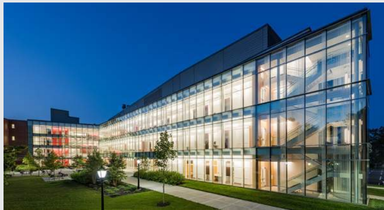
Glass Type II: CW with Vertical Line Ceramic Frit Pattern
