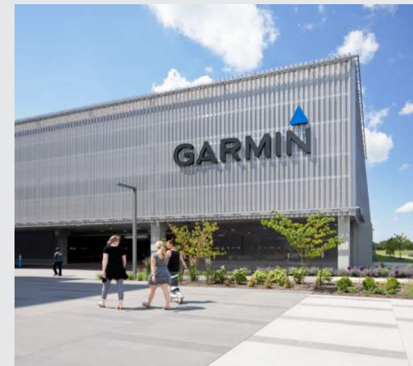
Perforated, Corrugated Stainless Steel Facade Screen
