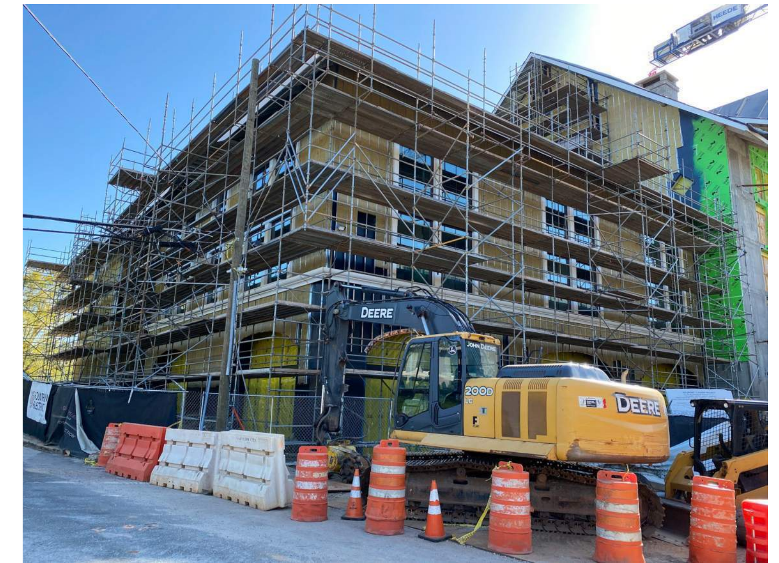
Construction progress of SE corner of Bohemian Hotel
