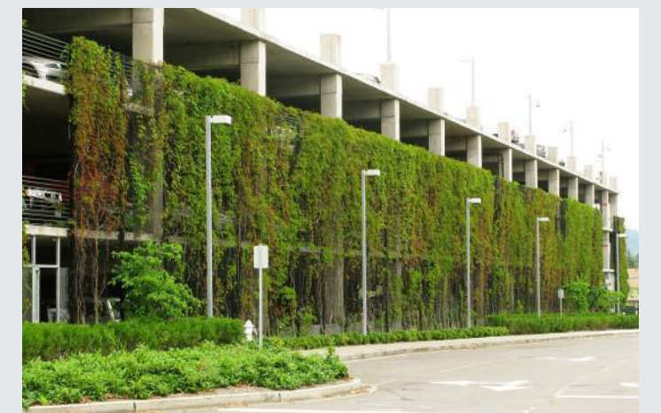
"Greenscreen" Modular Trellis - Falls St Elevation only
