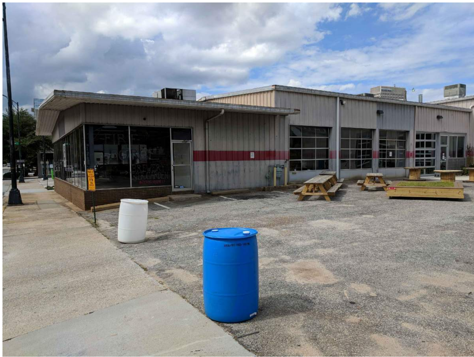
CONTEXT VIEW - EAST
