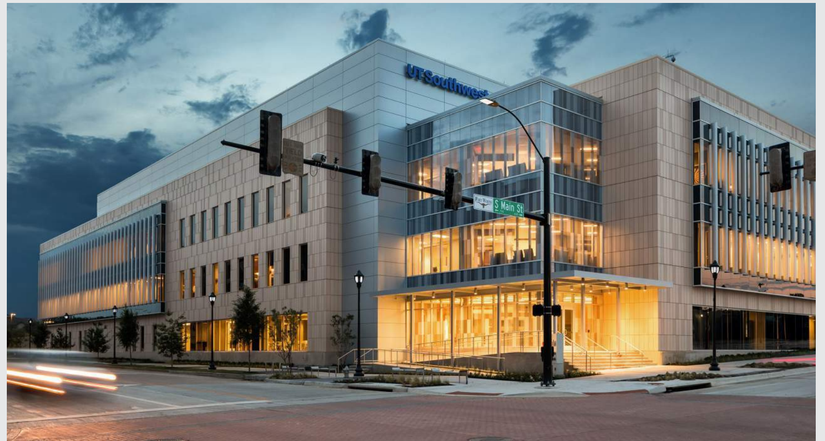
Extruded Clay Panelized Rainscreen
