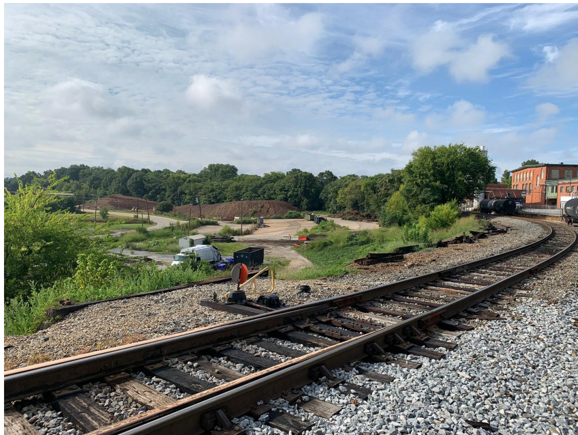
VIEW TO NORTH (FROM RAILWAY)
