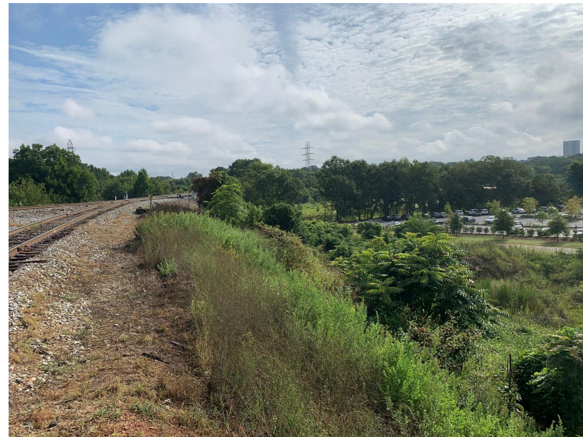
VIEW FROM RAILWAY TO MAYBERRY AND BRIDGE OVERPASS
