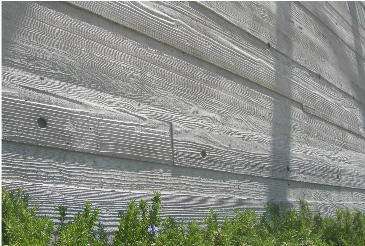
BOARD FORMED CONCRETE
