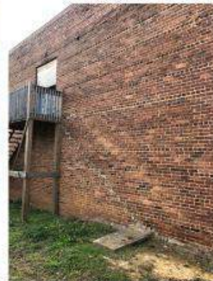
Original stairs went from Pendleton Street to upstairs. Now a wooden staircase leads up from the Burdette Street side of the building.
