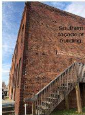
Bricks change from the eastern façade to the southern façade.
