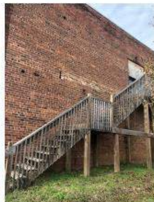
Staircase to second floor.
