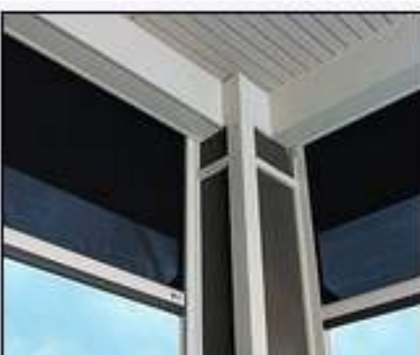
Wood Clad Column
