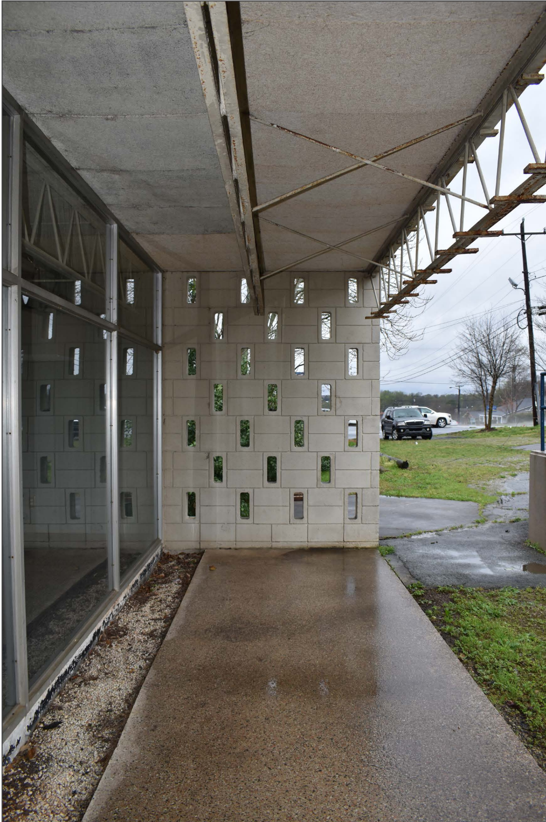
4. North elevation, main entrance detail including terrazzo, breeze-block and exposed structural members.
