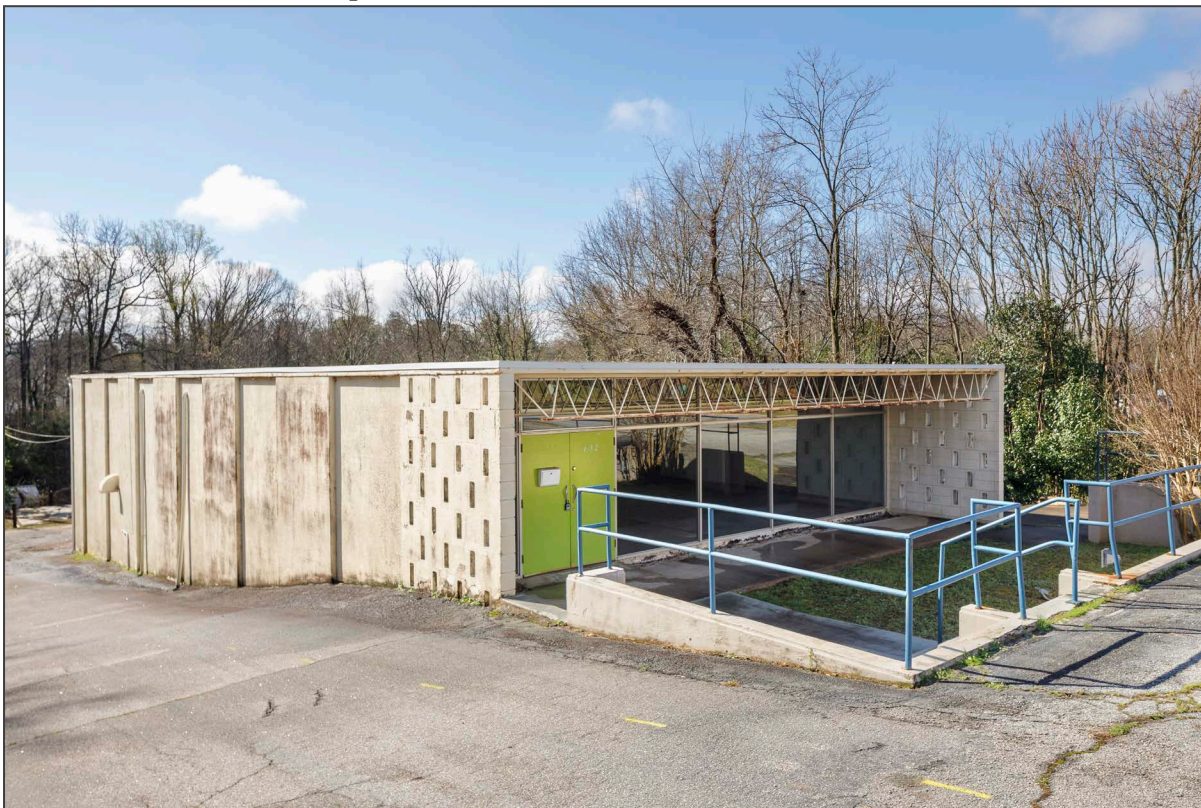
1. north and east elevations, view south. Copyright Kris Decker/Firewater Photography. Do not use without permission.
