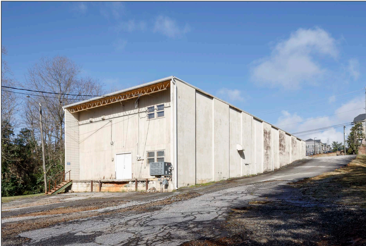
5. West and south elevations, view northwest. Copyright Kris Decker/Firewater Photography. Do not use without permission.
