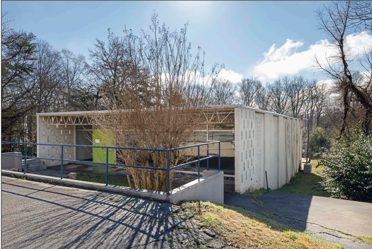
2. North and west elevations, view east. Copyright Kris Decker/Firewater Photography. Do not use without permission.
