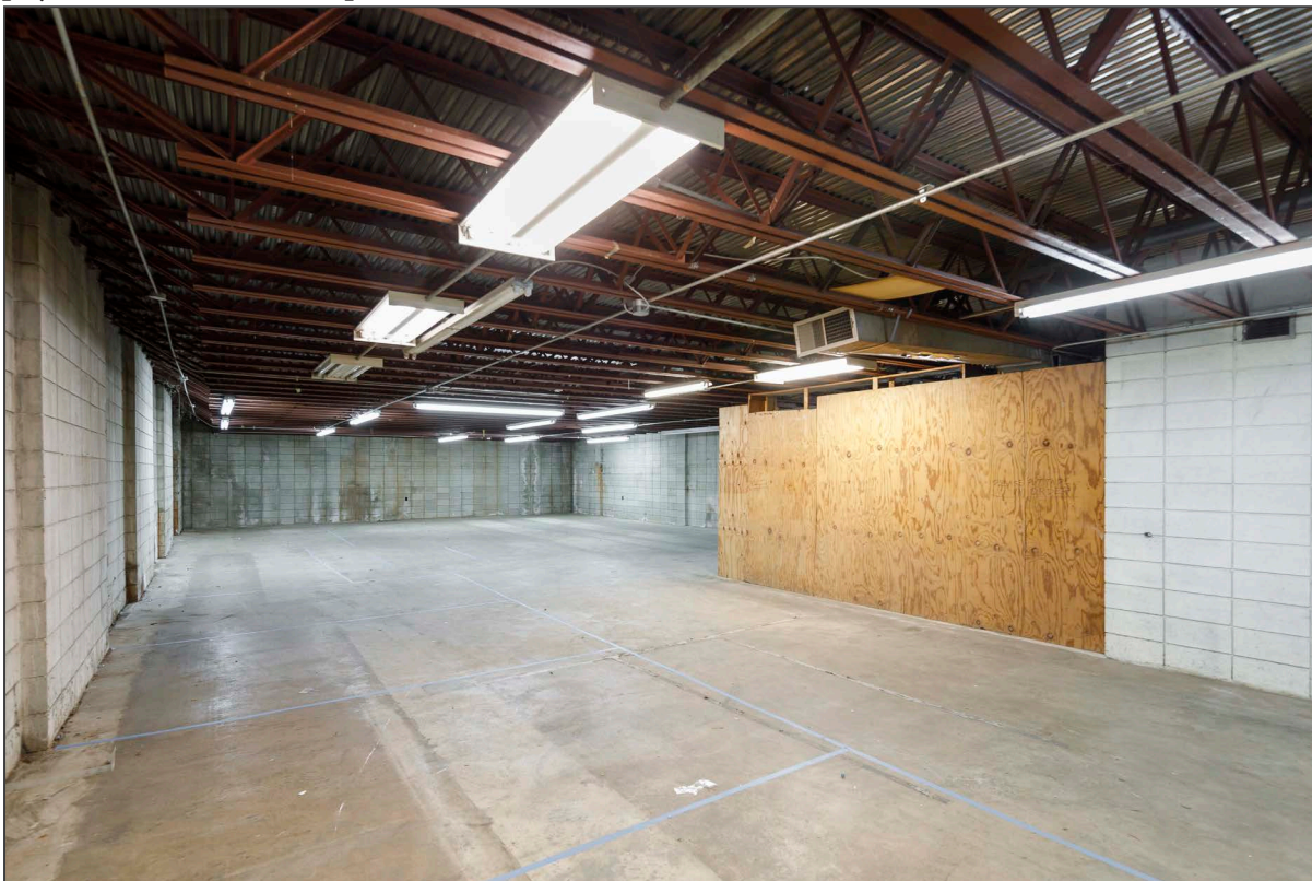
10. Basement, view north. Copyright Kris Decker/Firewater Photography. Do not use without permission.
