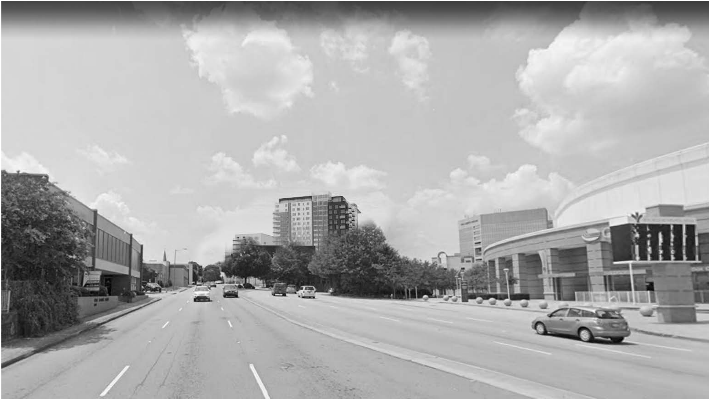
VIEW FROM E NORTH ST ON APPROACH
