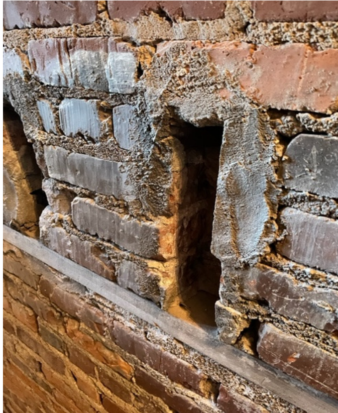
Existing Floor Framing Pocket at Interior Stair Addition
