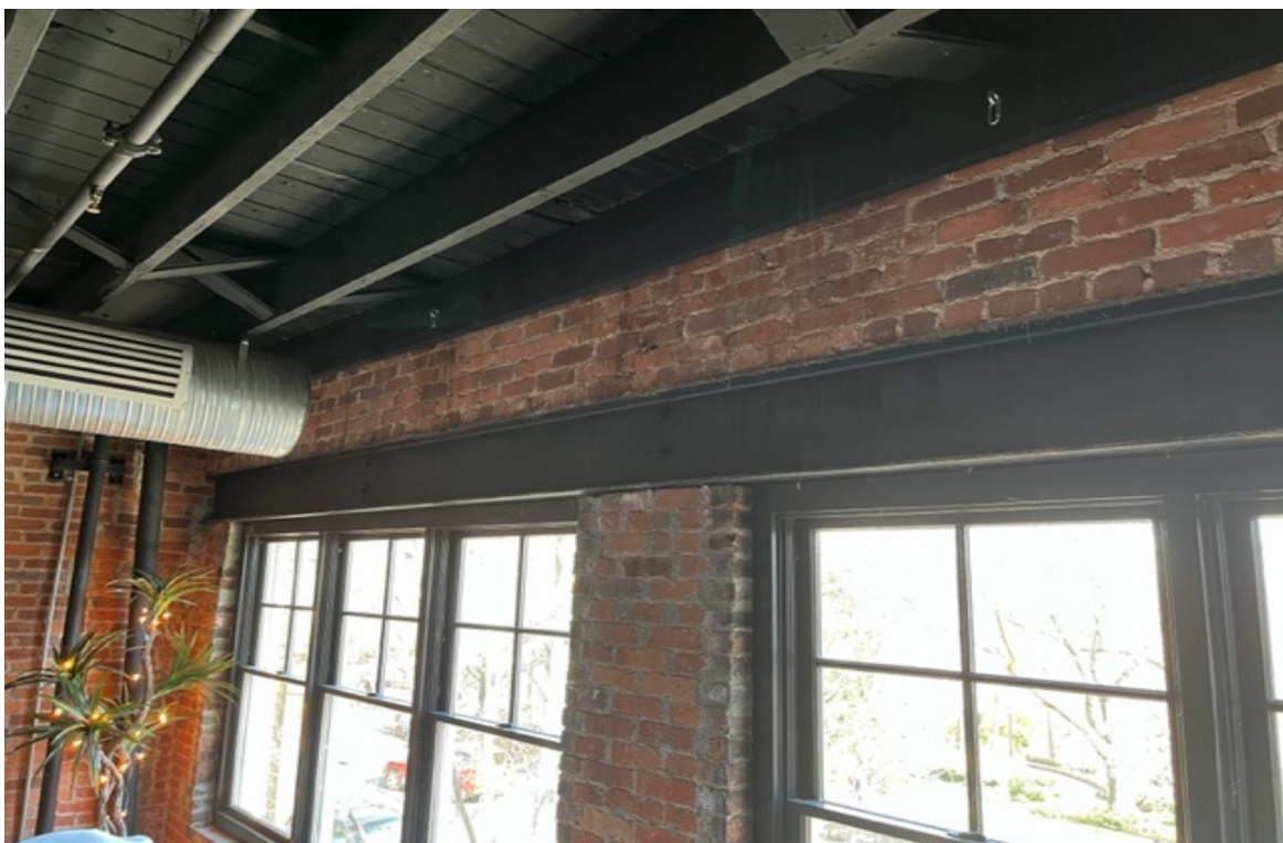
Existing Roof Framing and Residential Brick Header / Lintel
