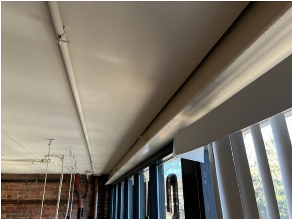
Existing Retail Storefront Brick Header / Lintel
