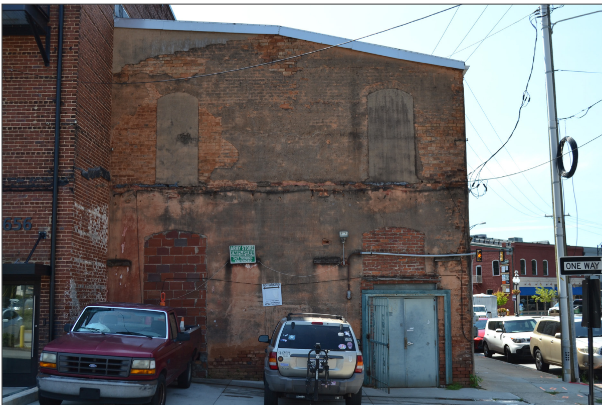
Image 15. North elevation, view south
