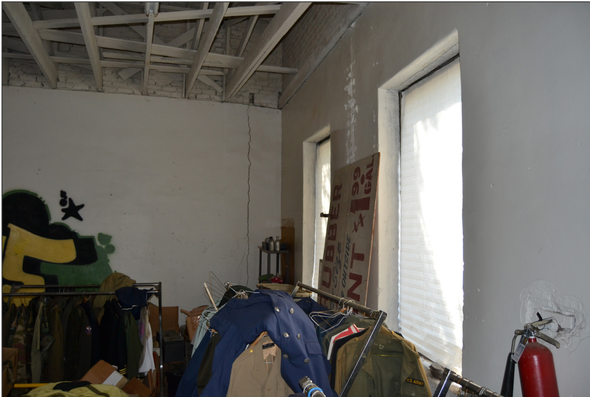
Image 31. Second floor, front room, view east
