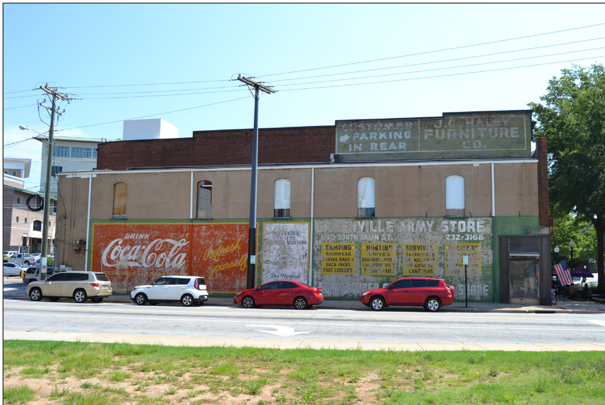
Image 11. West elevation, view east
