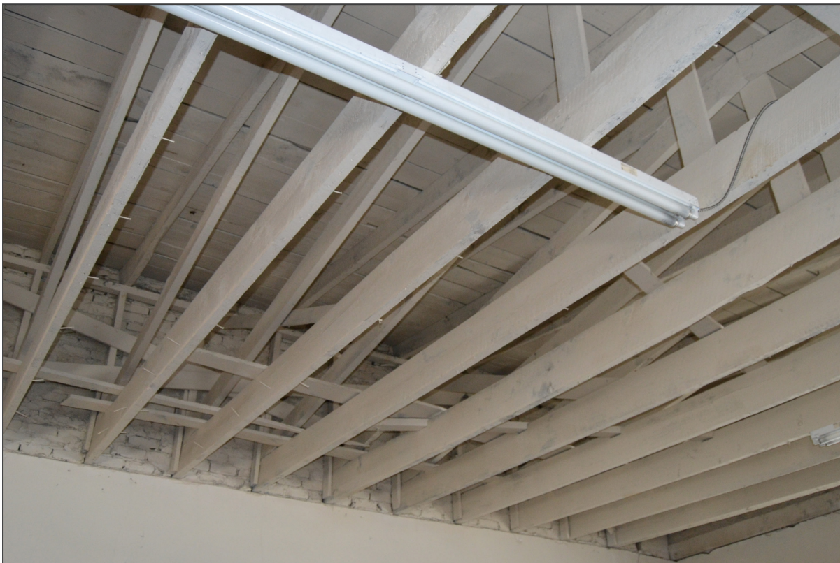
Image 34. Second floor, front room, rafter example
