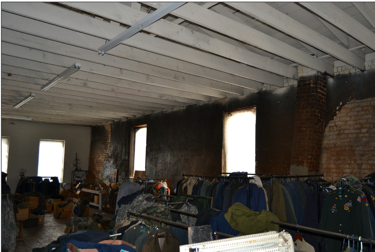
Image 30. Second floor, front room, view southwest
