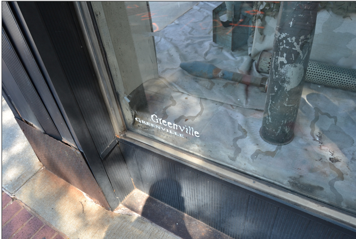
Image 10. South elevation, storefront, framing detail
