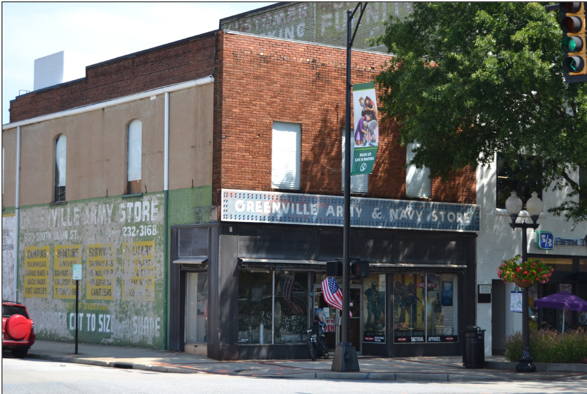
Image 4. South elevation, view northeast
