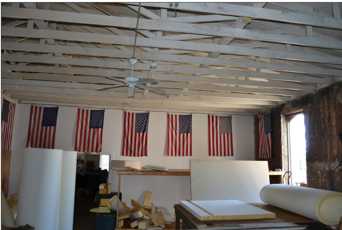
Image 24. Second floor, rear room, view south
