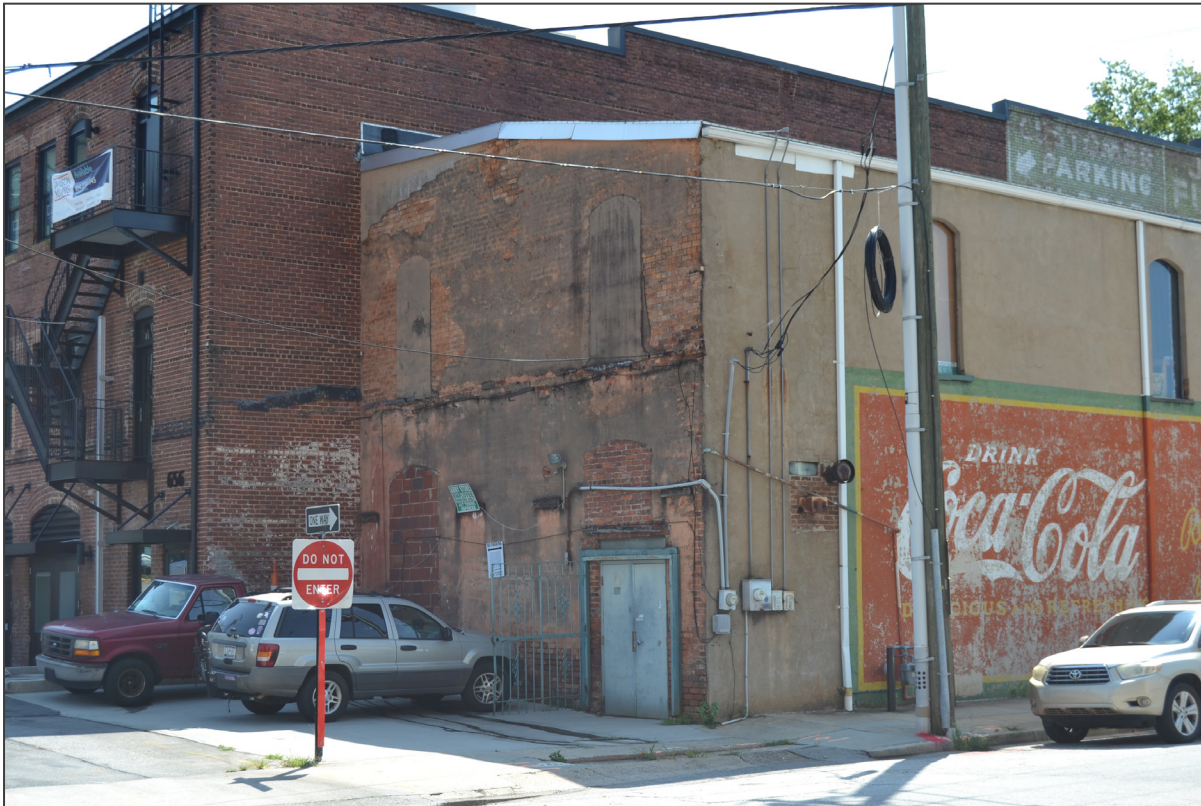
Image 14. North and west elevations, view southeast
