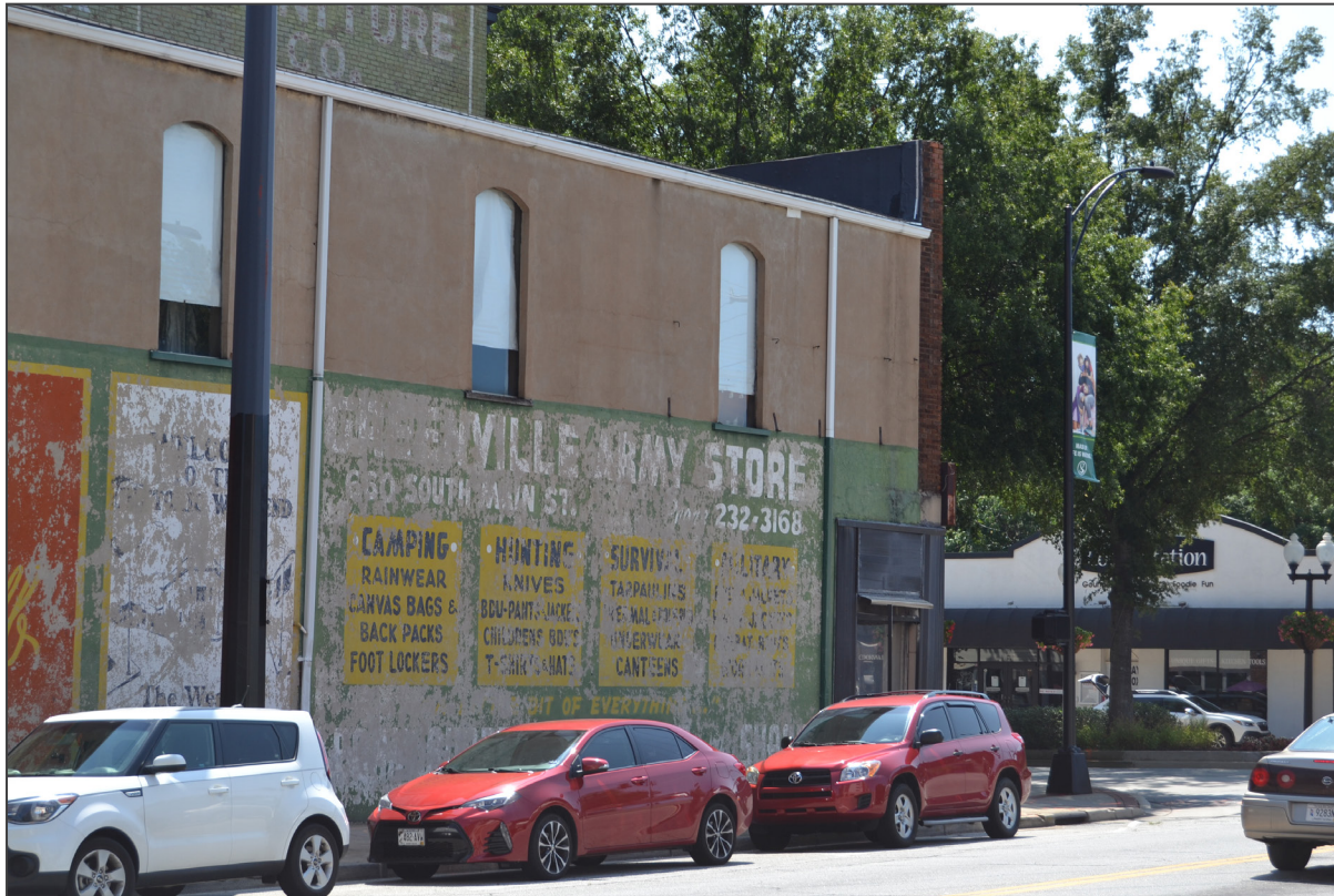
Image 12. West elevation, view southeast
