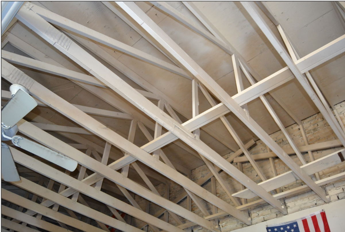
Image 27. Second floor, rear room, exposed roof rafters
