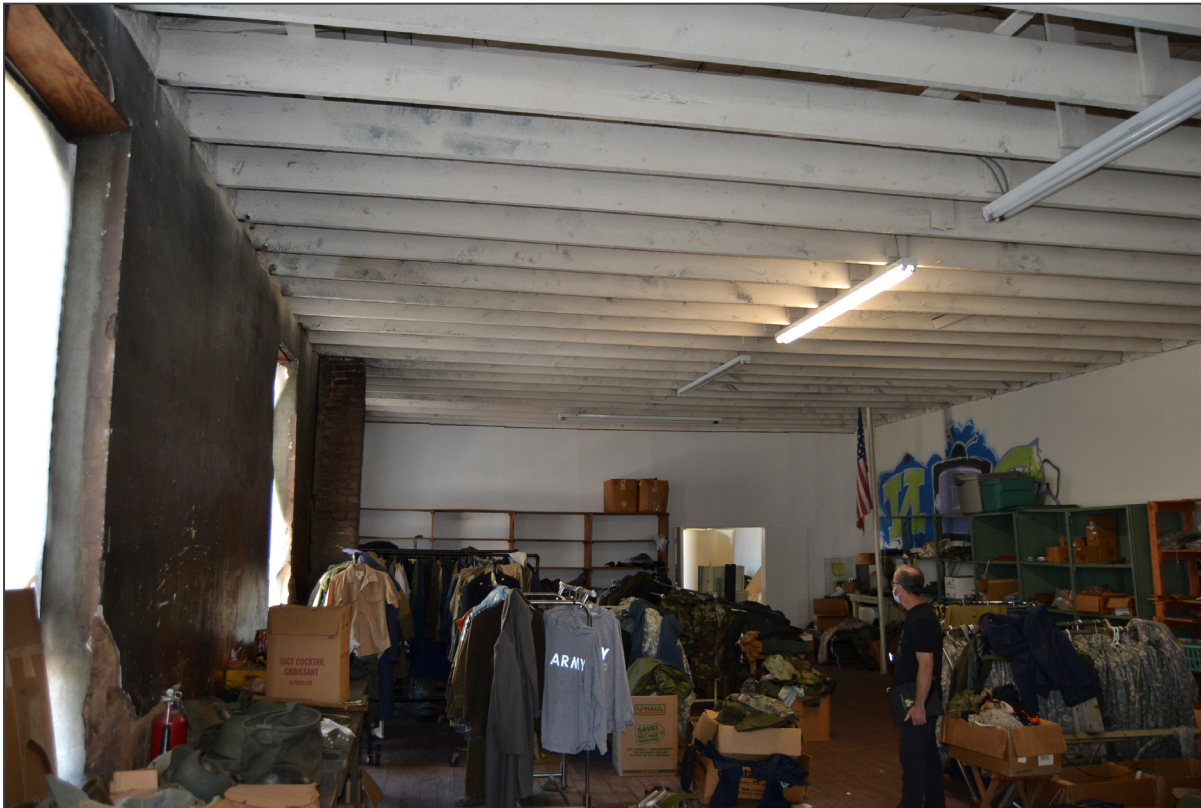
Image 29. Second floor, front room, view north
