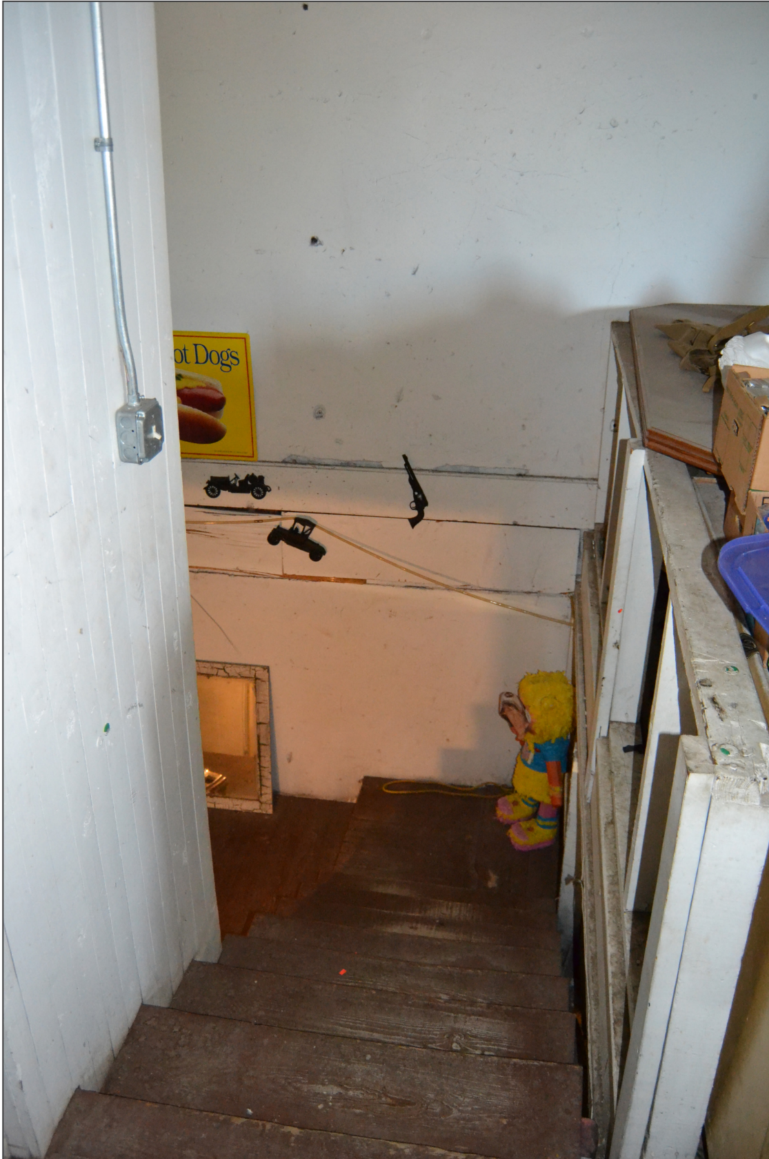
Image 22. Second floor, view north
