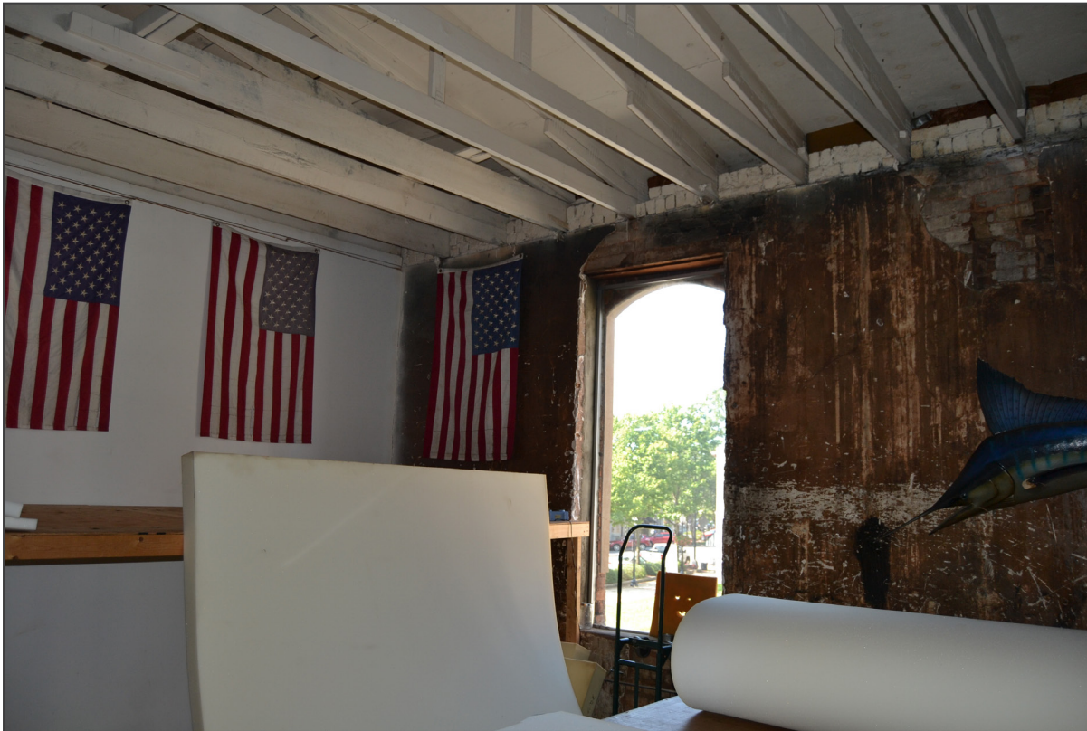
Image 25. Second floor, rear room, view southwest
