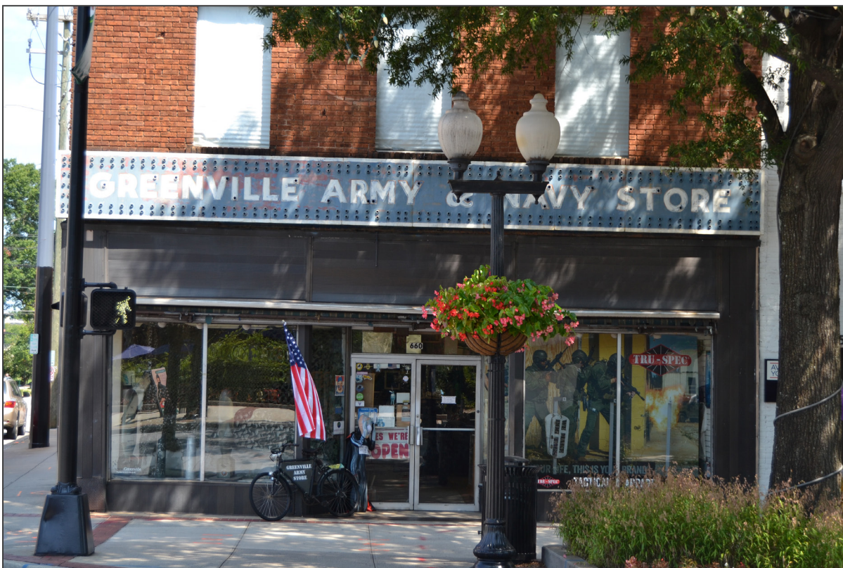
Image 5. South elevation, view north
