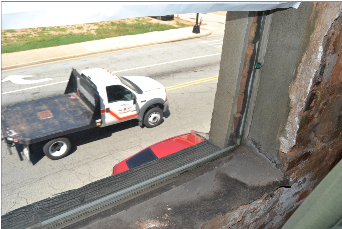
Image 32. Second floor, west window frame example
