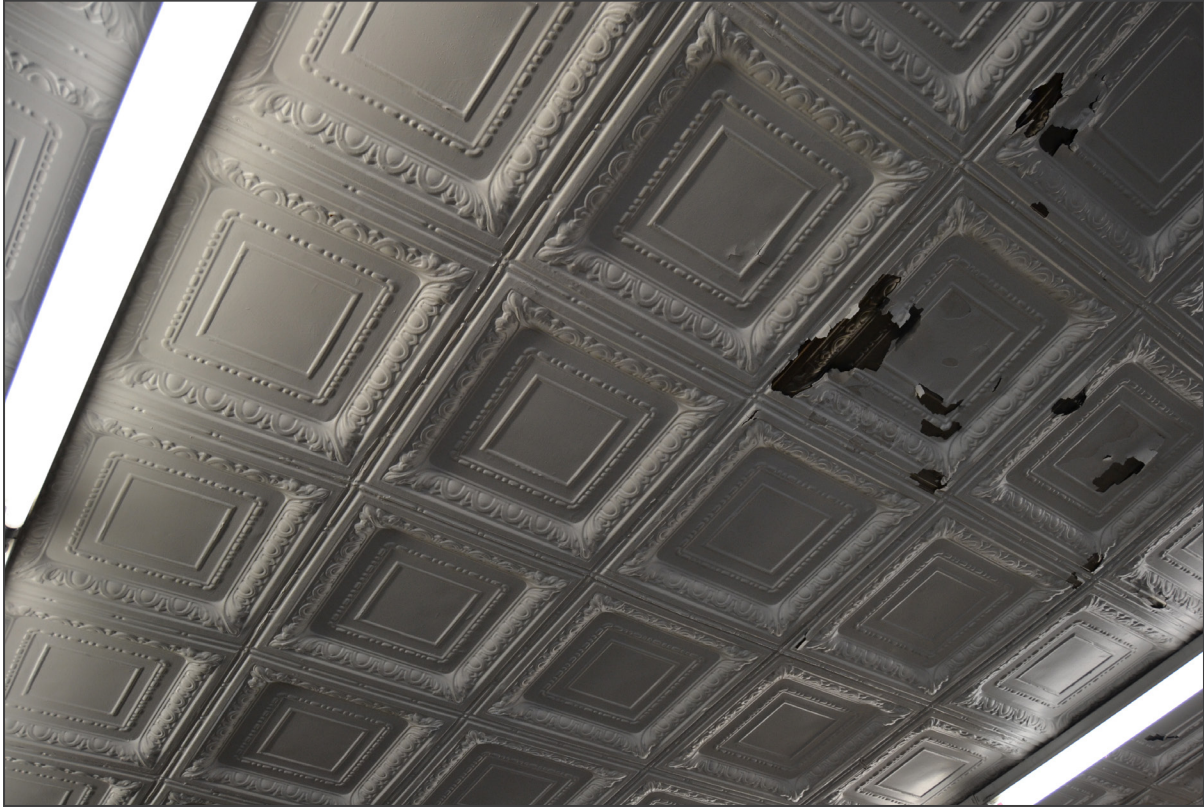
Image 18. First floor, historic pressed metal ceiling
