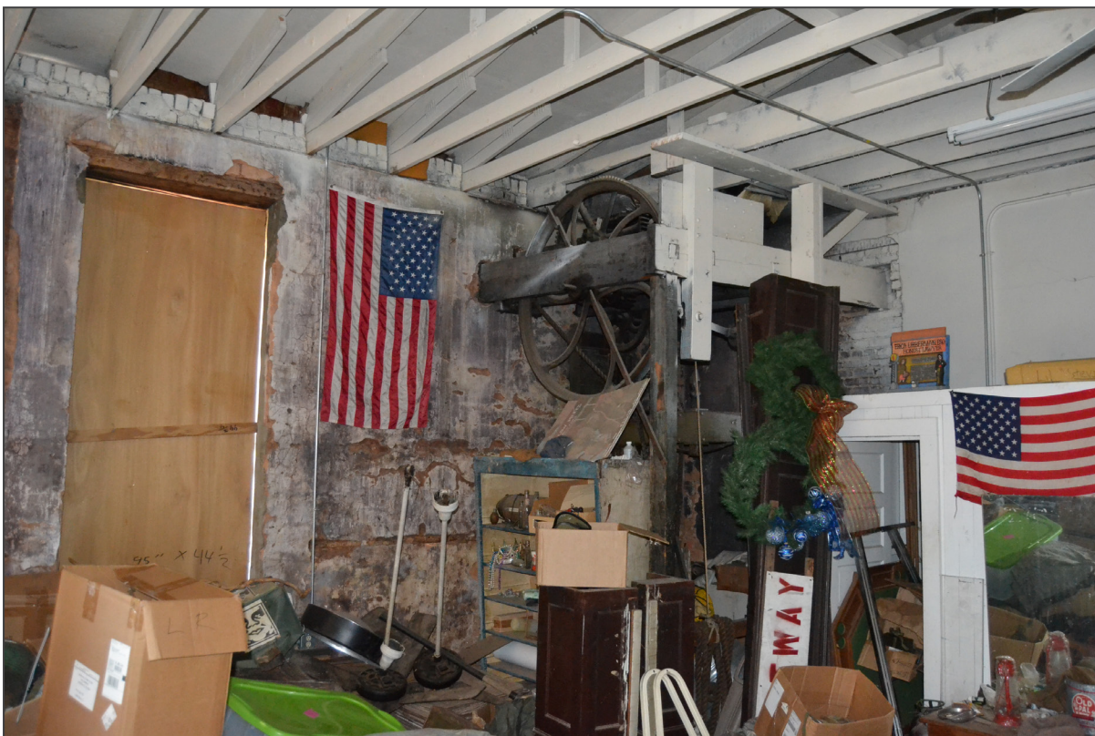
Image 26. Second floor, rear room, view northwest
