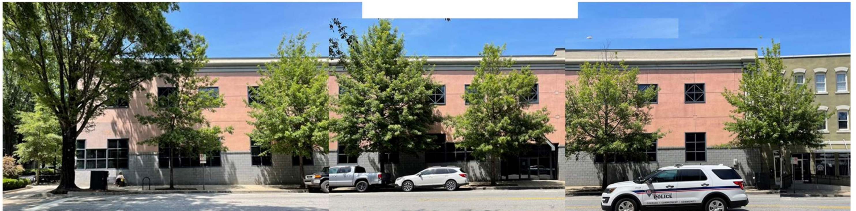
W. Washington Street (South) Facade
