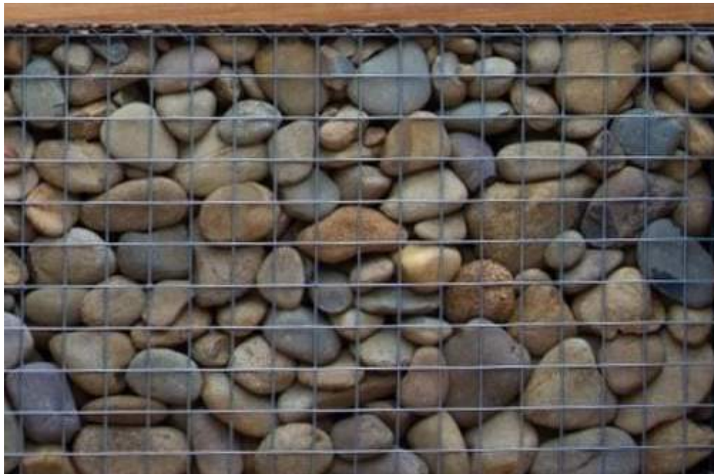
GABION SITE WALL + FENCE
