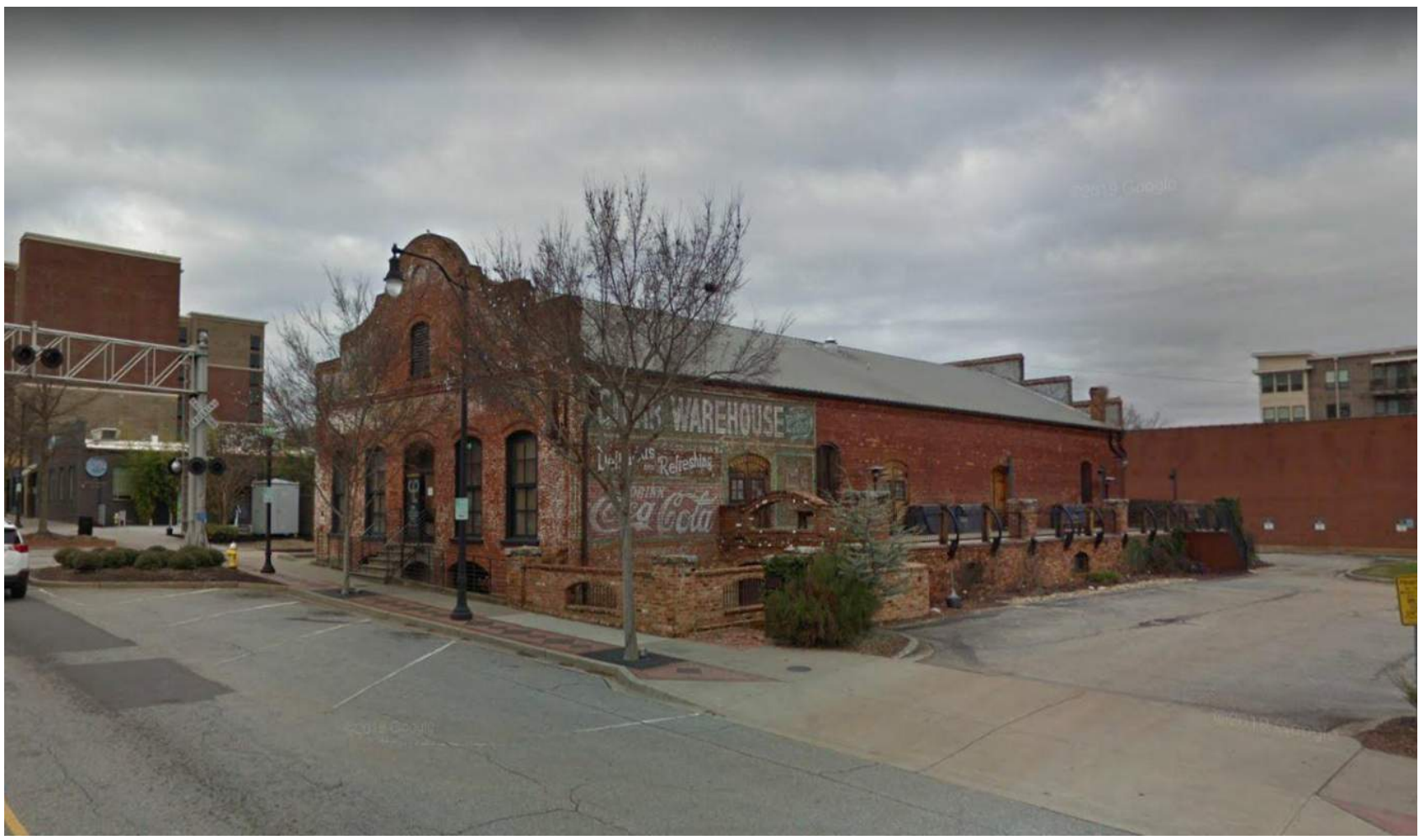
2 - VIEW OF EXISTING CIGAR WAREHOUSE FROM SOUTH MAIN STREET
