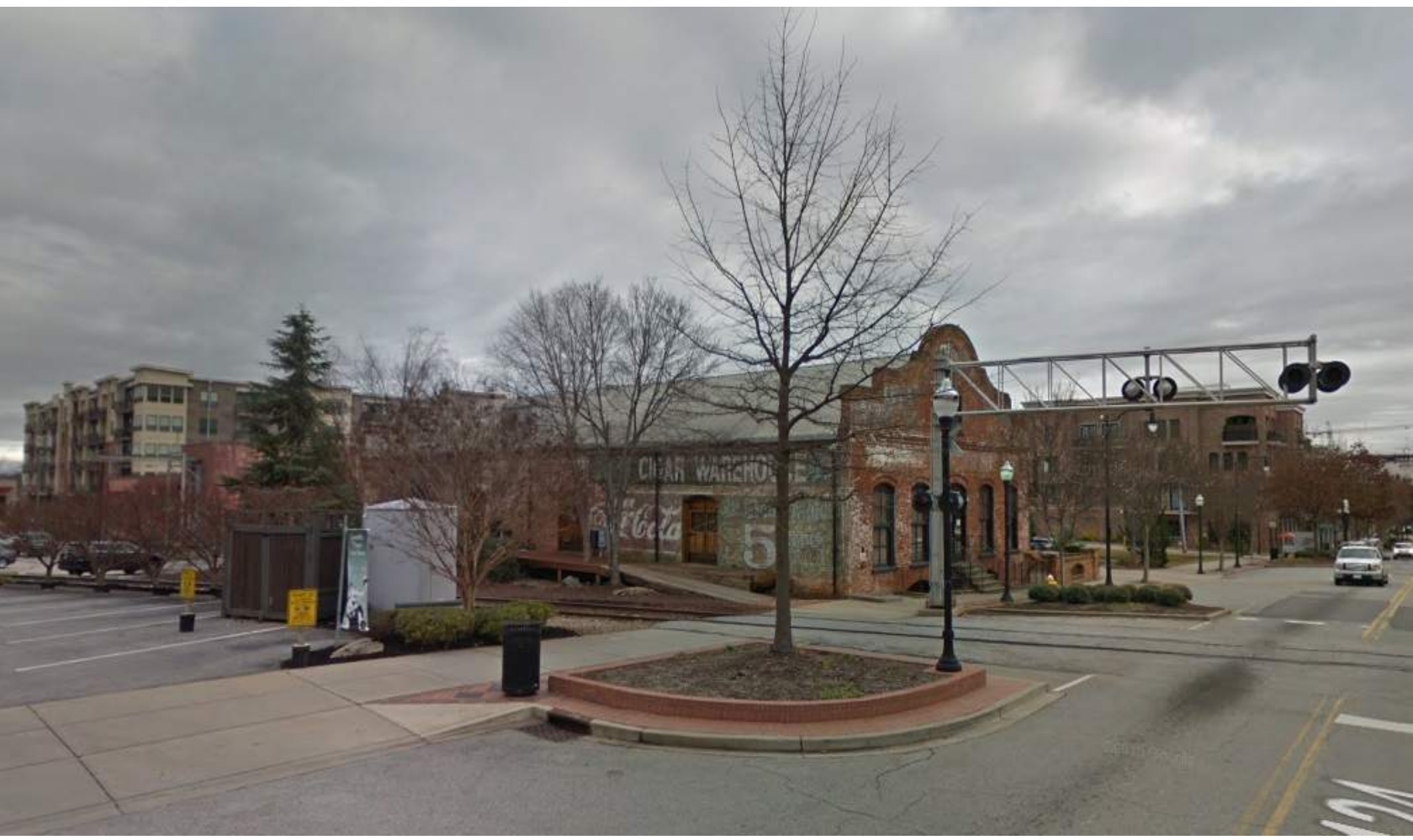
3 - VIEW OF EXISTING CIGAR WAREHOUSE FROM SOUTH MAIN STREET
