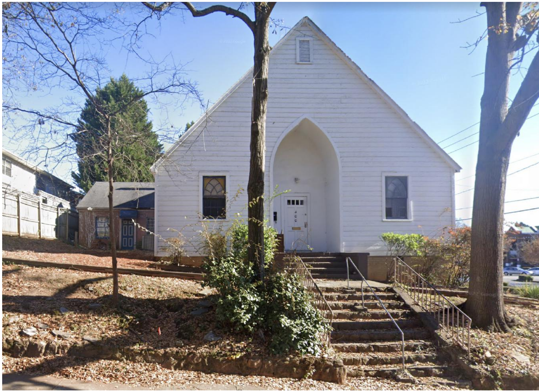
EXISTING WEST FACADE
