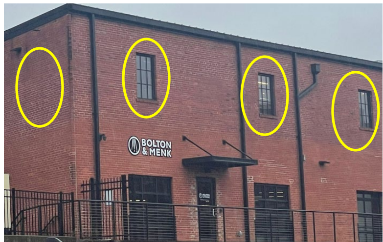
Existing Conditions – Window Locations
