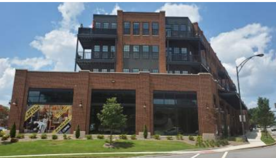
Loft Construction on Buncombe Rd, Greenville, SC
