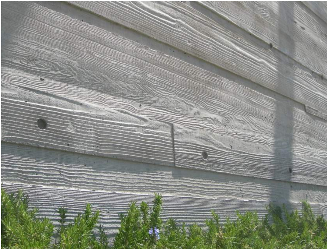
BOARD FORMED CONCRETE
