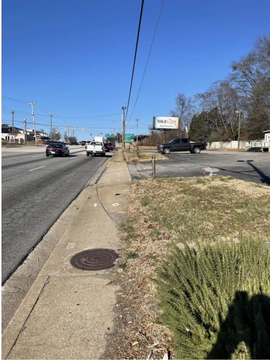
PROJECT SITE ALONG PLEASANTBURG DRIVE FACING NORTH
