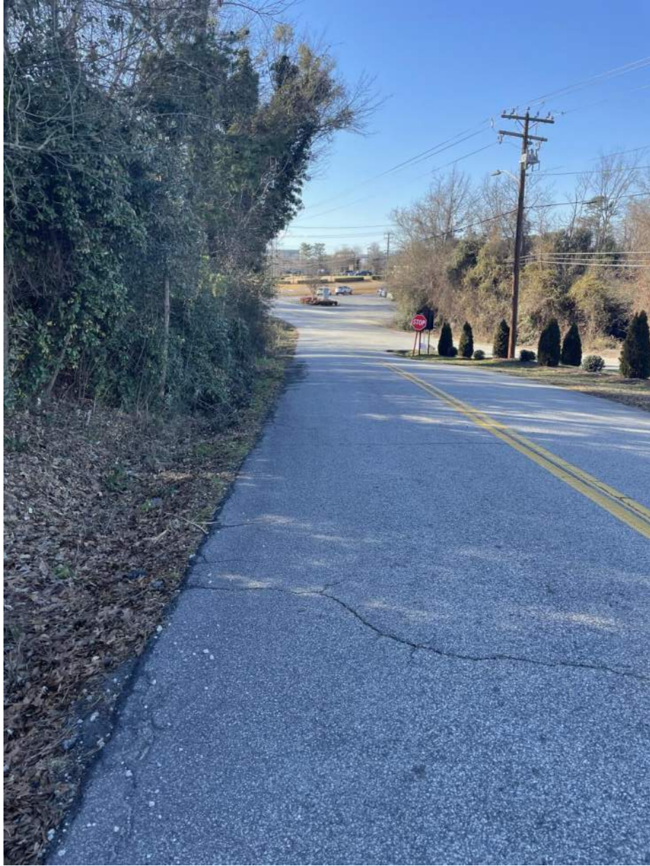
PROJECT SITE ALONG WATSON AVIATION ROAD FACING WEST
