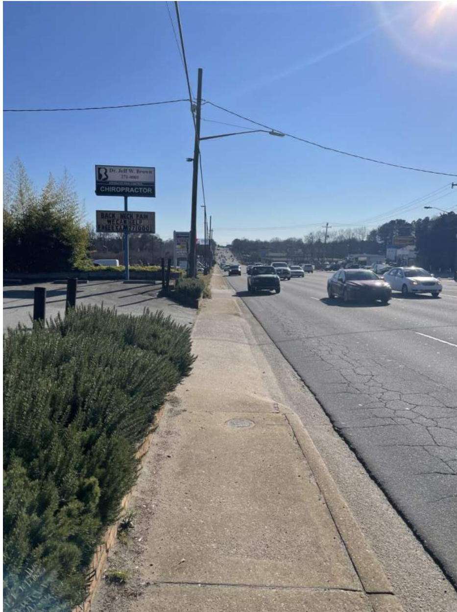
PROJECT SITE ALONG PLEASANTBURG DRIVE FACING SOUTH
