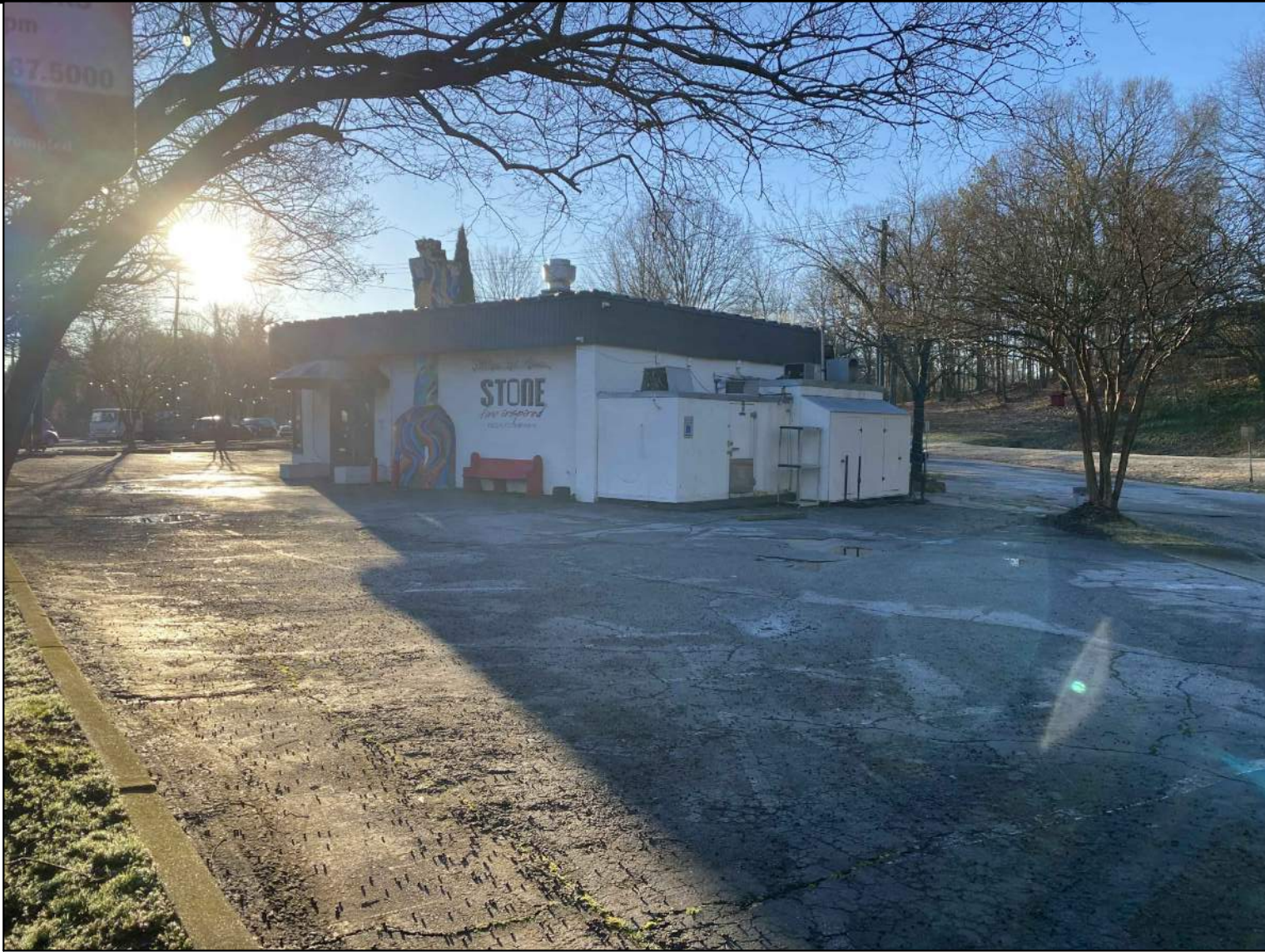
EXISTING RESTAURANT (EAST OF PROPOSED DEVELOPMENT)
