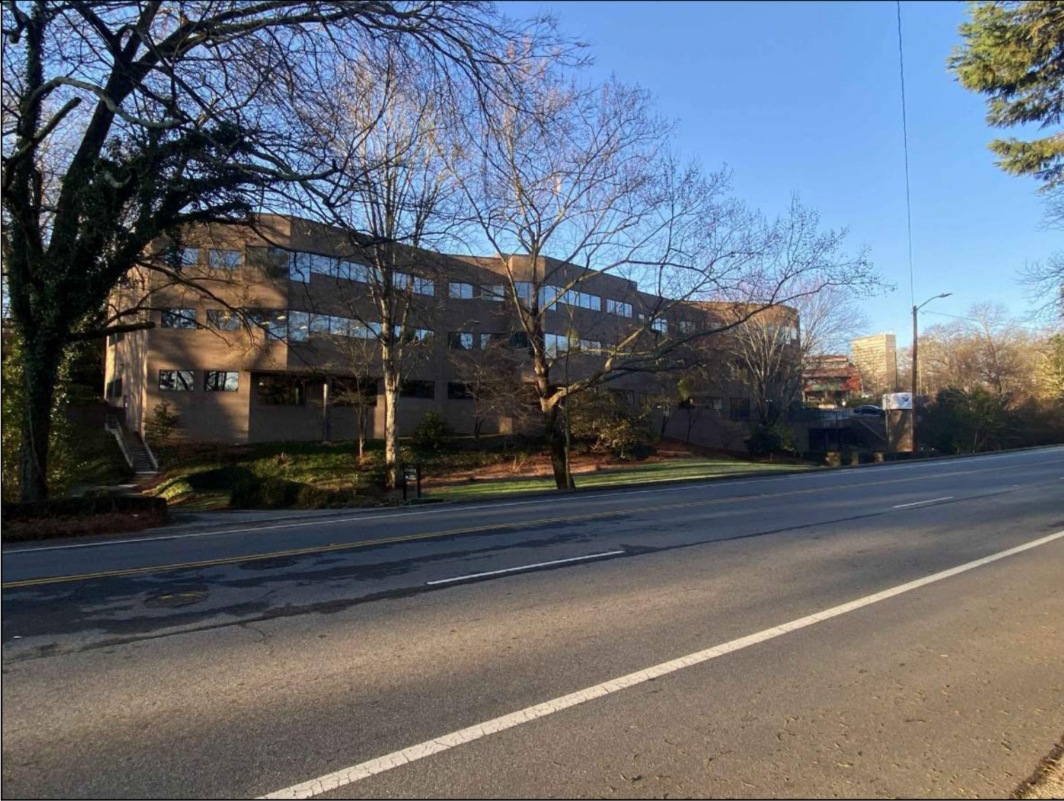
EXISTING OFFICE BUILDING (WEST OF PROPOSED DEVELOPMENT)
