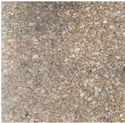
EXISTING AGGREGATE PANELS
