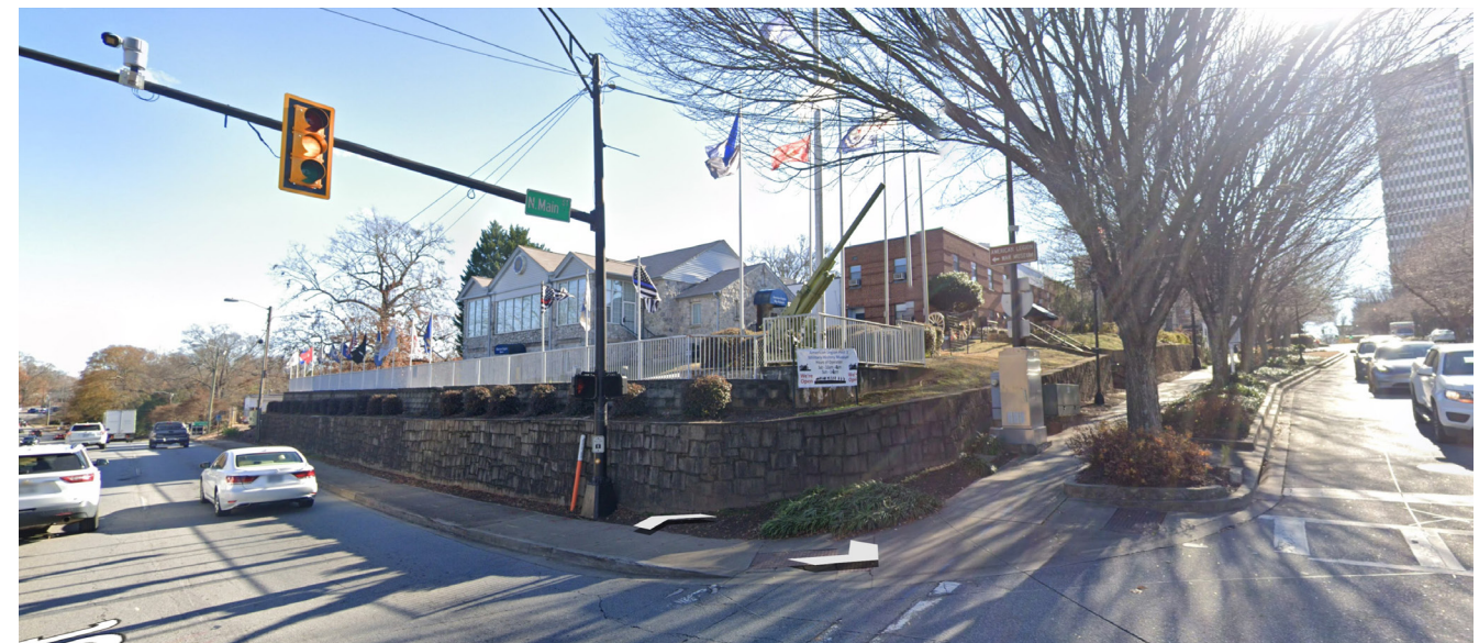
View of site from intersection of Academy and Main Street
