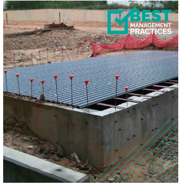
Figure 10-5-4. Typical Underground Detention Vault
