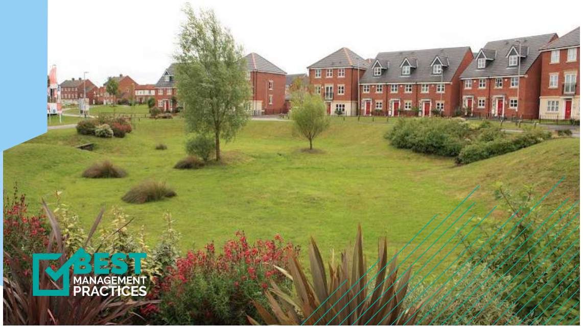
Figure 10-5-1. Typical Dry Detention Basin
