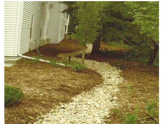
Figure 10-6-8. Typical Infiltration Trench.
