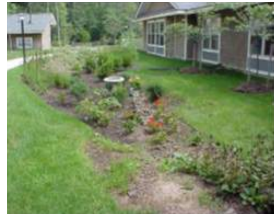
Figure 10-6-4. Typical Bioretention Basin.
