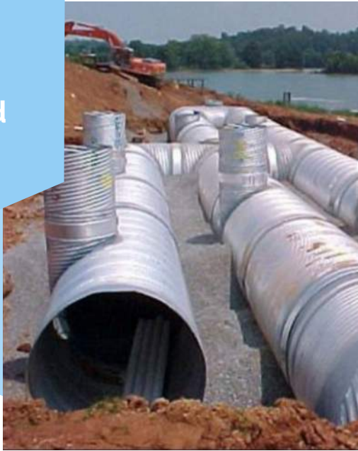
Figure 10-5-3. Typical Underground Large Pipe Detention System
