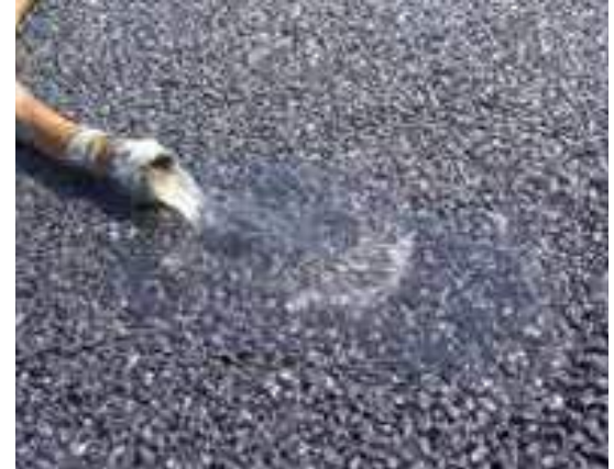
Figure 10-6-5. Typical Porous Asphalt.
