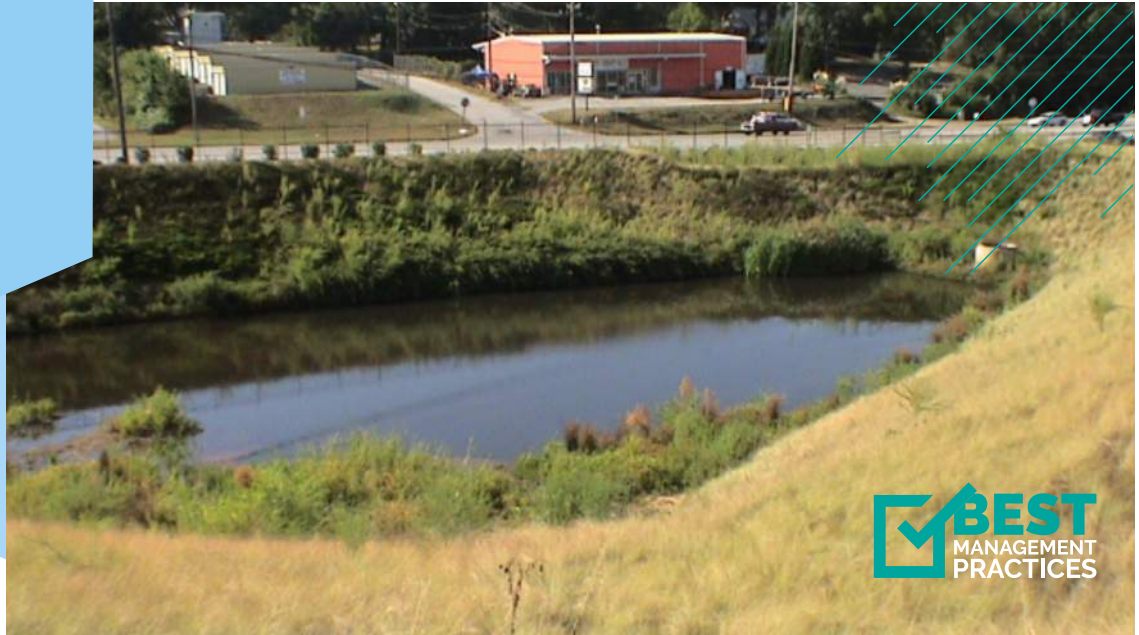
Figure 10-5-2. Typical Wet Detention Basin
