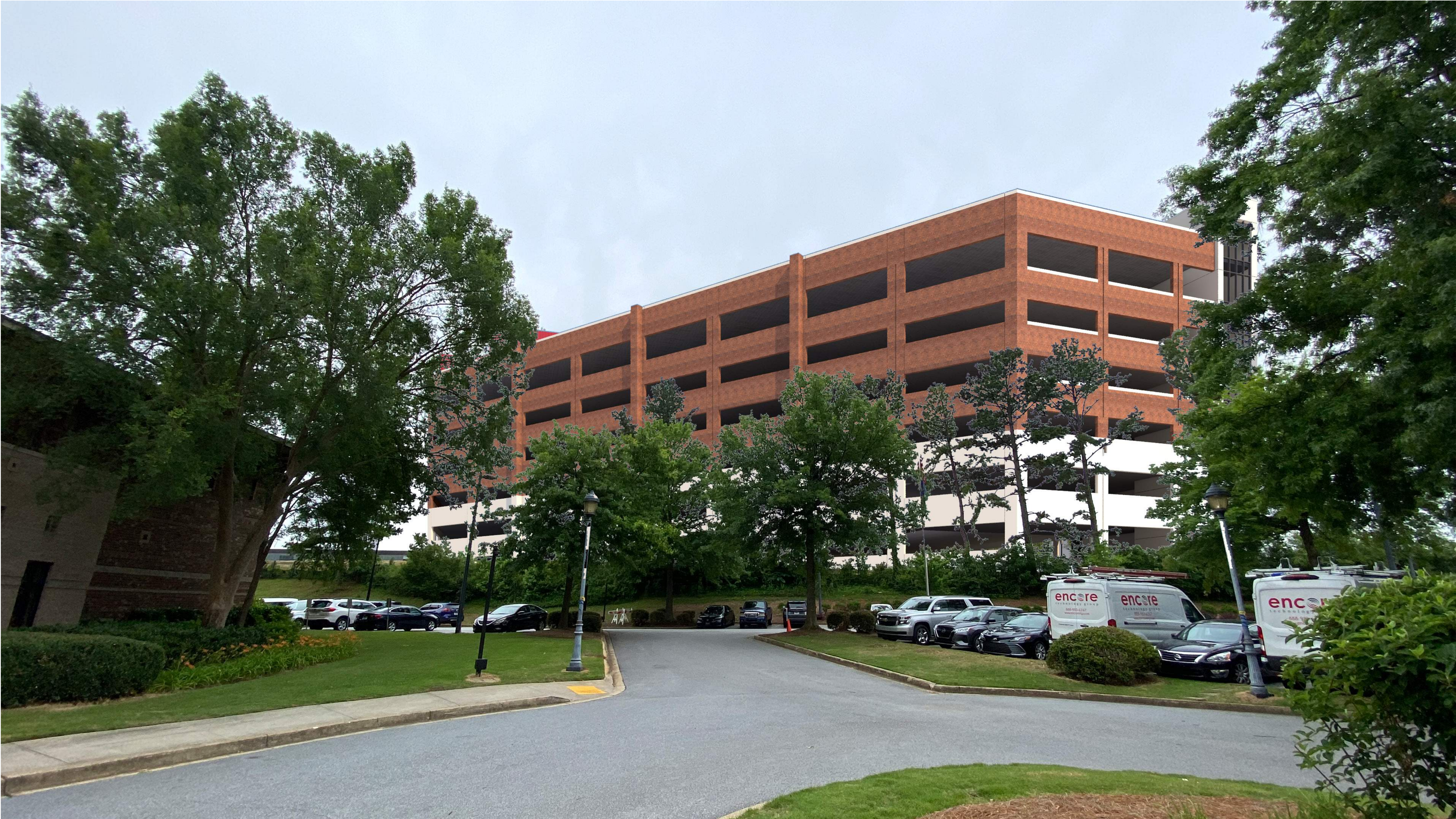
(E) Exterior view from Governor’s school parking I
