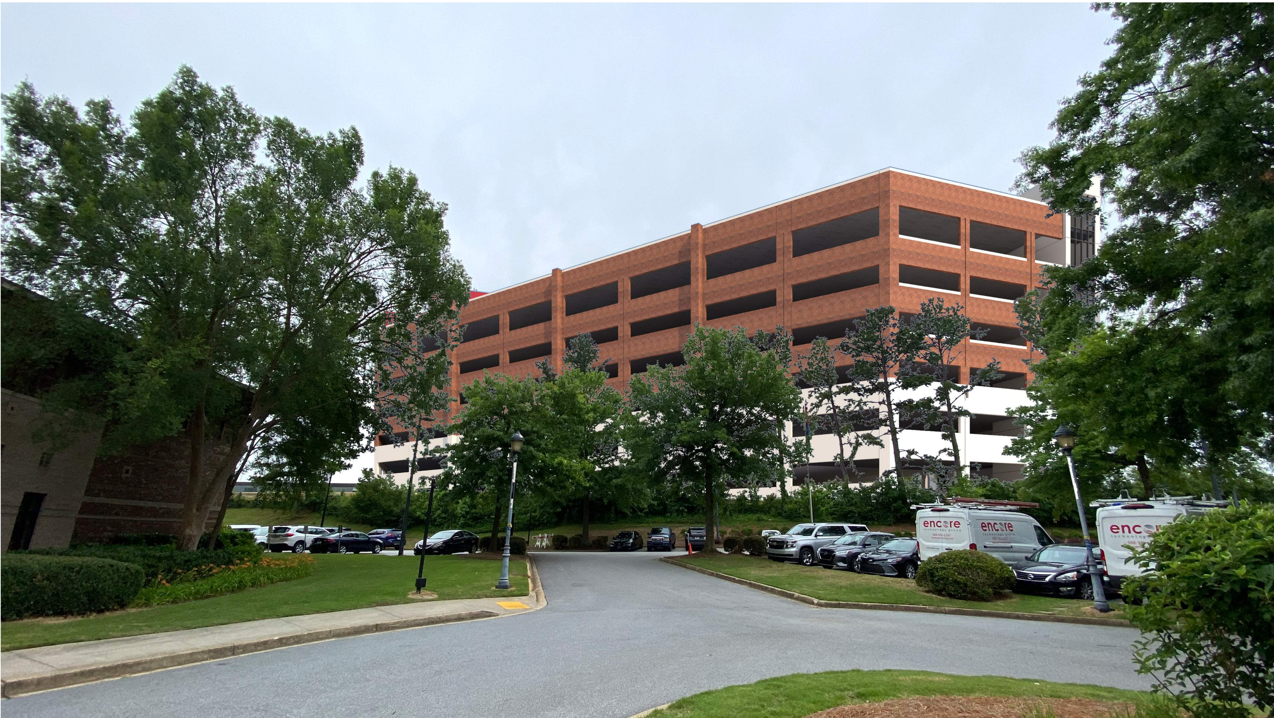
(E) Exterior view from Governor’s school parking I
