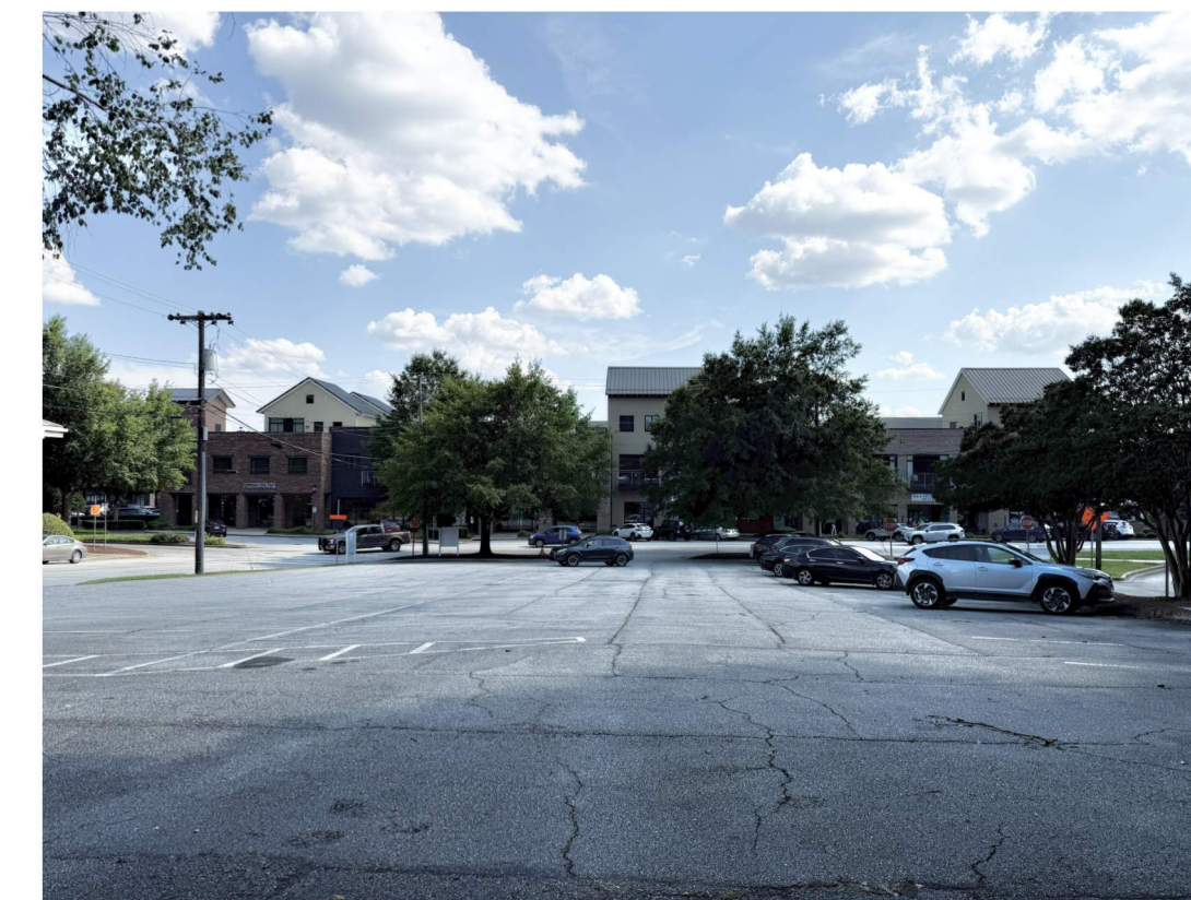
5 VIEW SOUTH FROM REAR OF PARCEL
