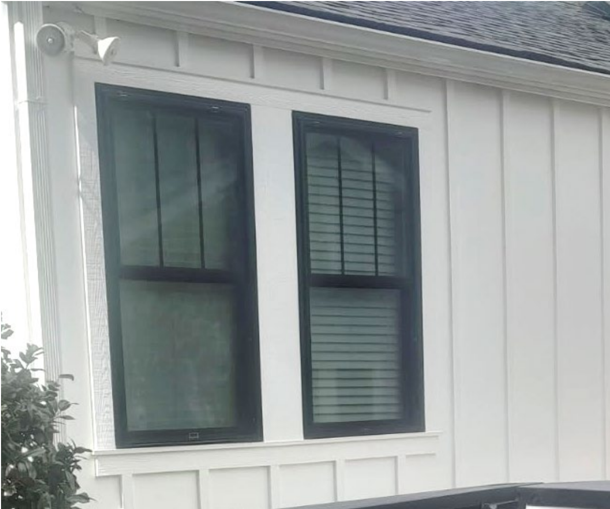
Windows black double hung with vertical grids in top sash, no grids in bottom (pella or equal).
