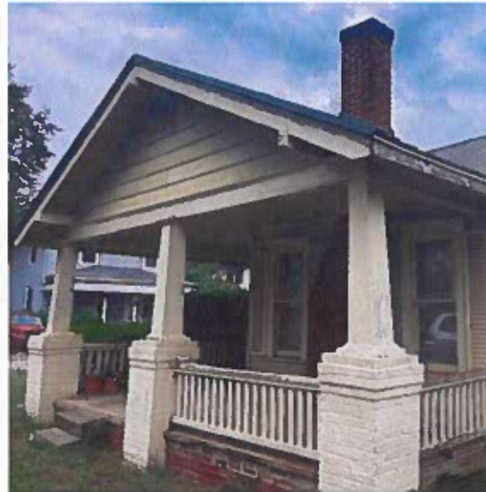
Side Porch Conditions
