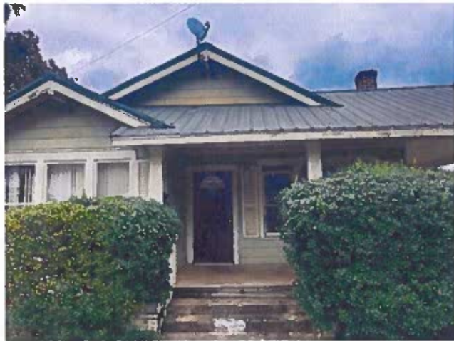
Existing Front Conditions
