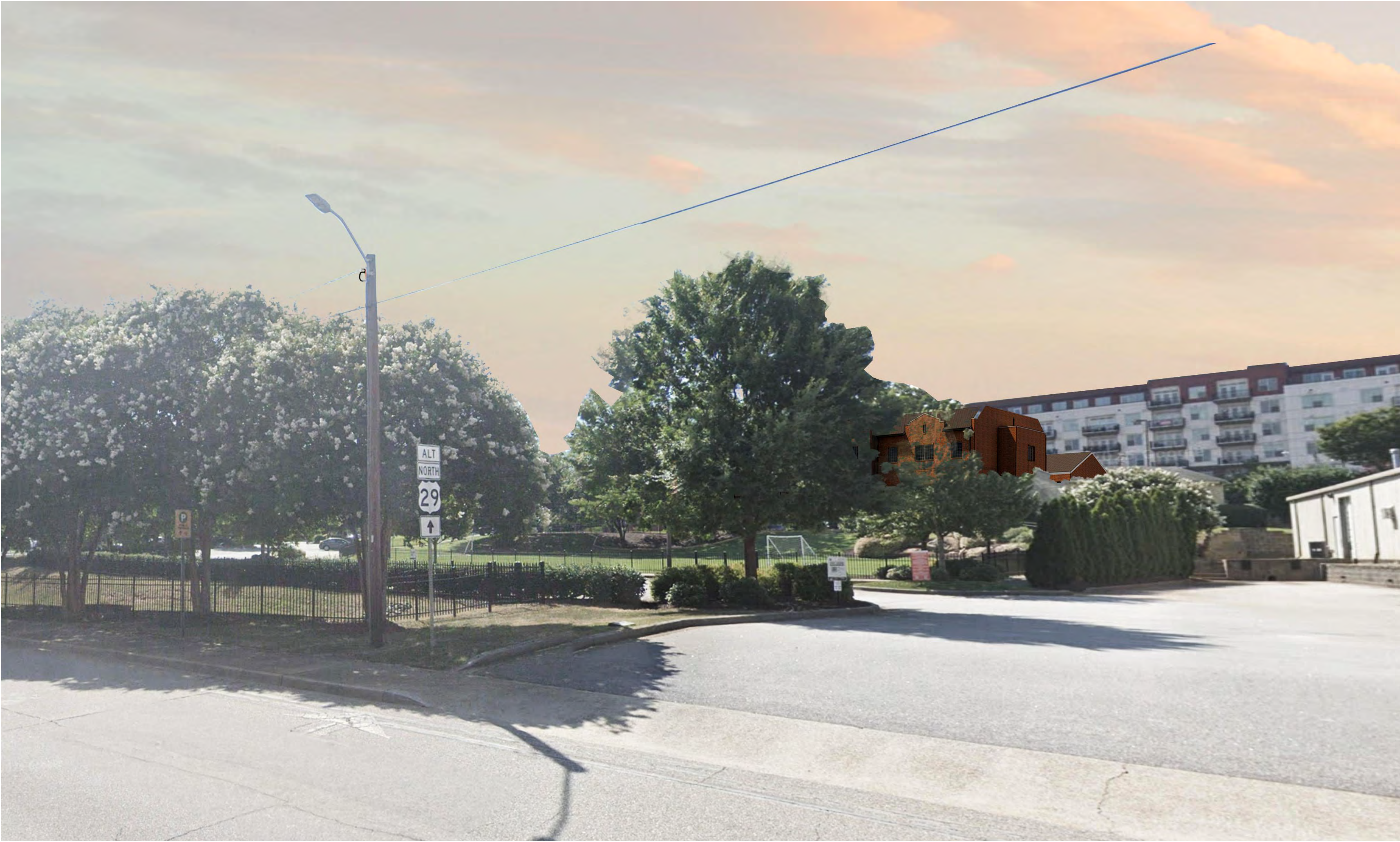
VIEW FROM ACADEMY STREET
