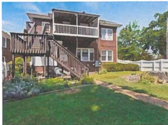
Rear Elevation: View from backyard
