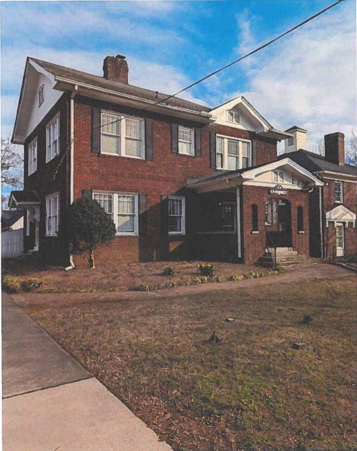
Front Elevation: View from corner of N. Main St. & Earle St.
