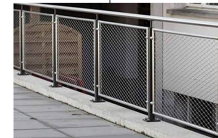
10. MESH PANEL RAILING
