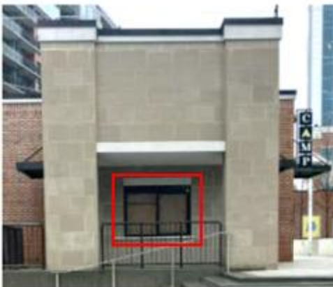
Existing Windows to be replaced
