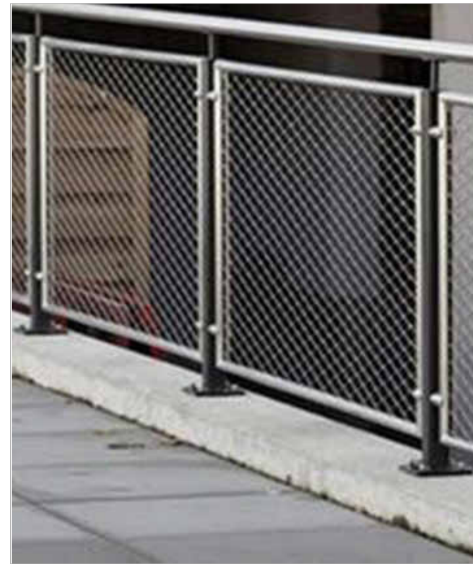
10 METAL RAILING + MESH PANELS
