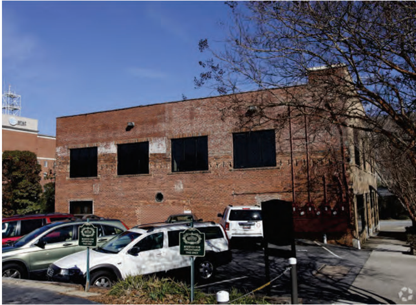
Photo 5: Side view of property
