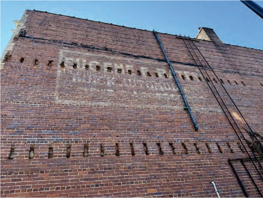
Photo 6: Street side view of property with original paint signage
