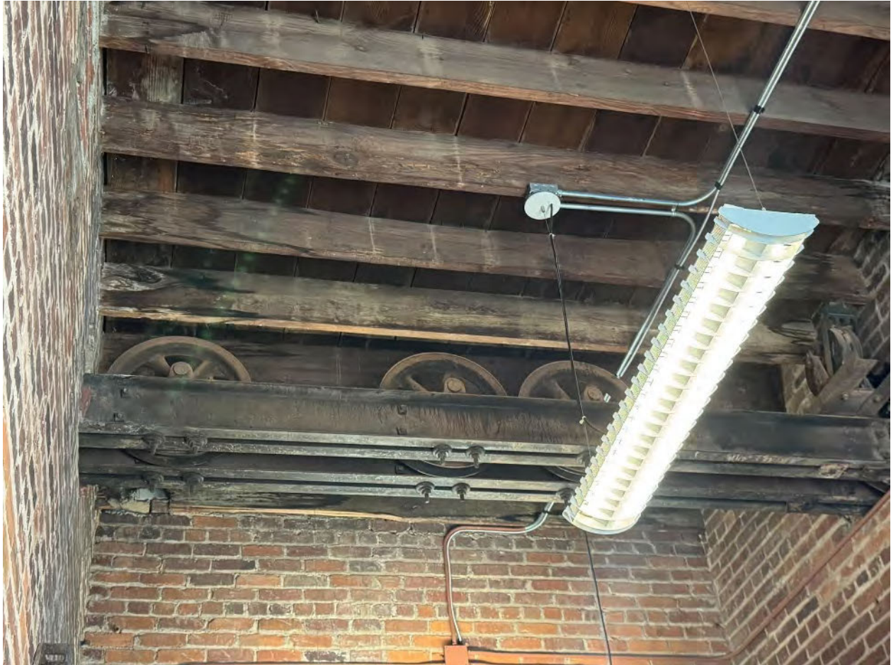
Original pulley system
