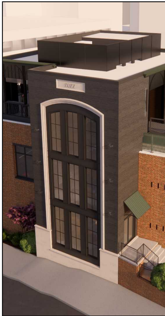
STAIR TOWER GIVES ACCESS TO ALL LEVELS OF THE BUILDING
