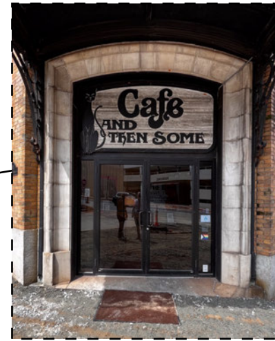
PRECAST AT MAIN ENTRANCE OF BUILDING
