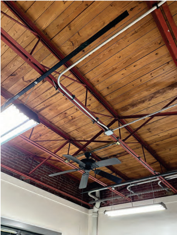
Photo 18: Original office space ceiling
