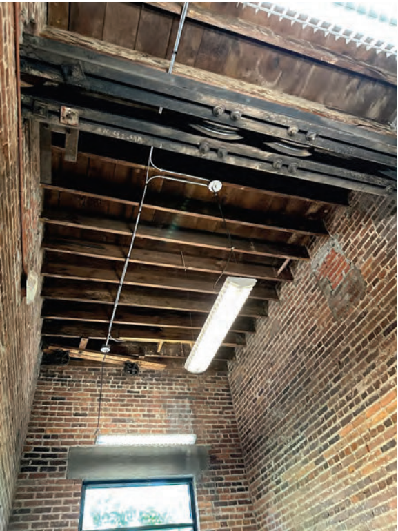
Photo 16: Pulley system in stairwell, close up
