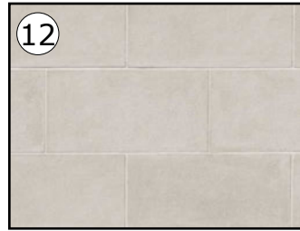
Stair Tower Window Surround: Material: Sto-Cast Finish: Cut limestone to match base material
