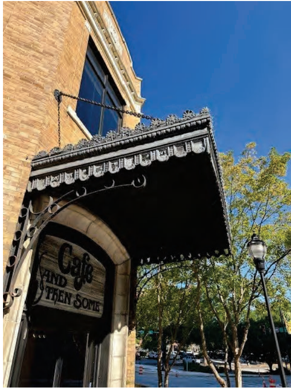
Photo 3: Original metal awning side view
