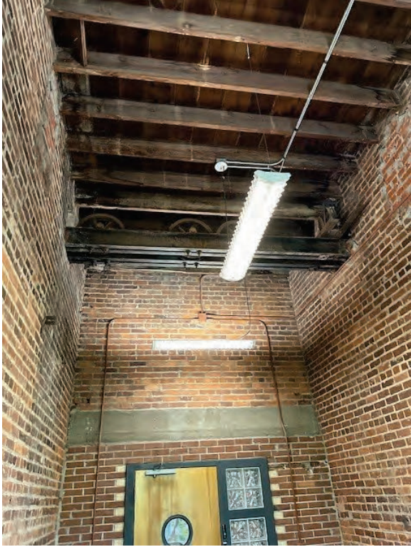
Photo 15: Pulley system in stairwell
