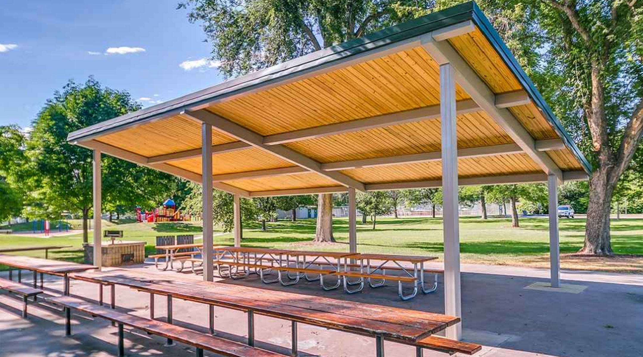
MONOSLOPE STAGE COVERING
