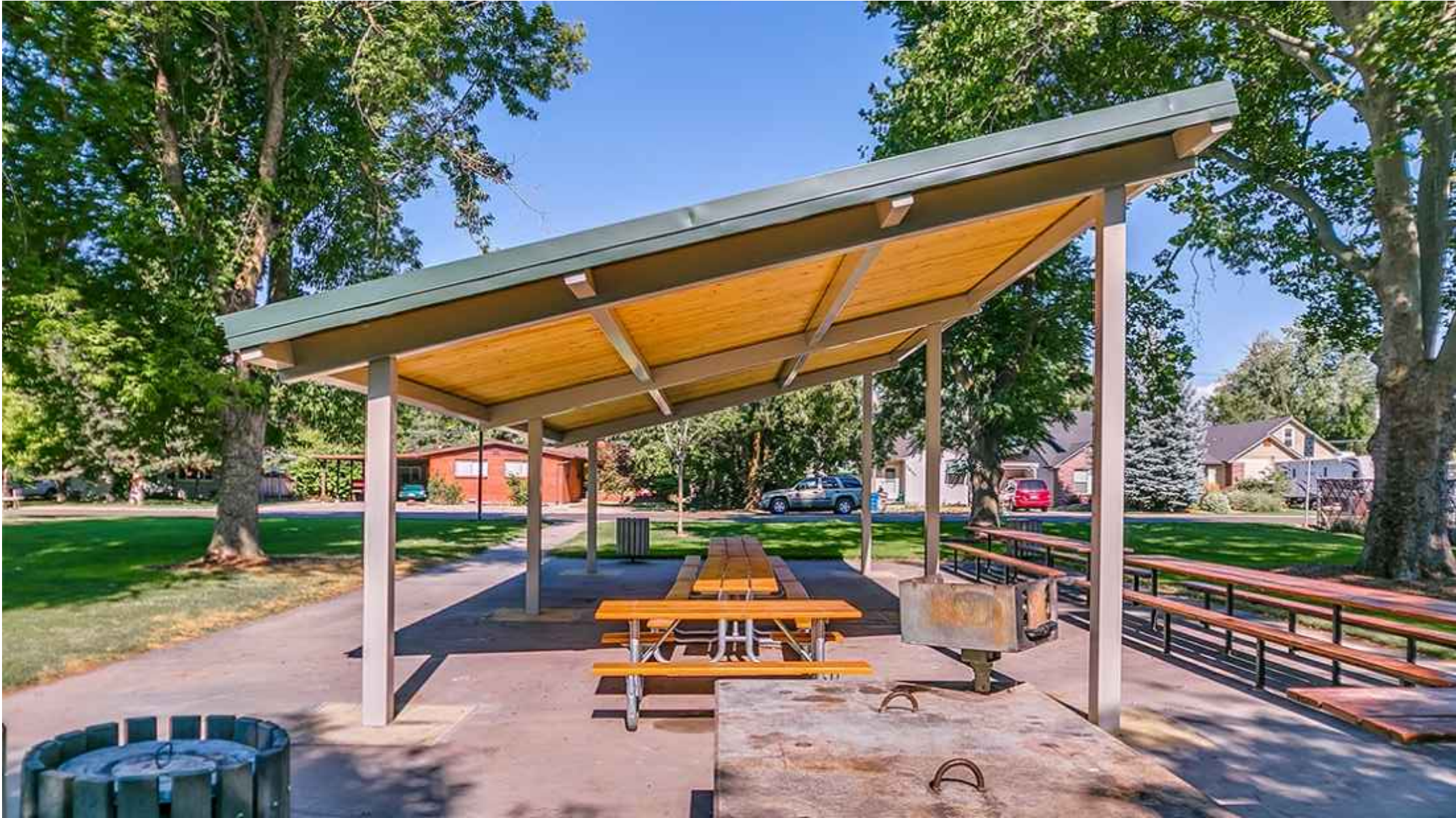
MONOSLOPE STAGE COVERING
