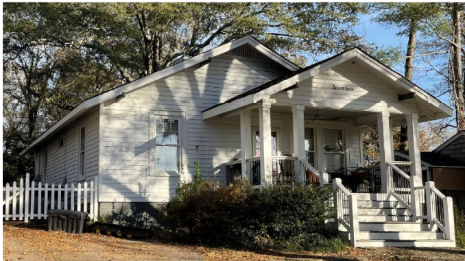
Current Façade Photo
