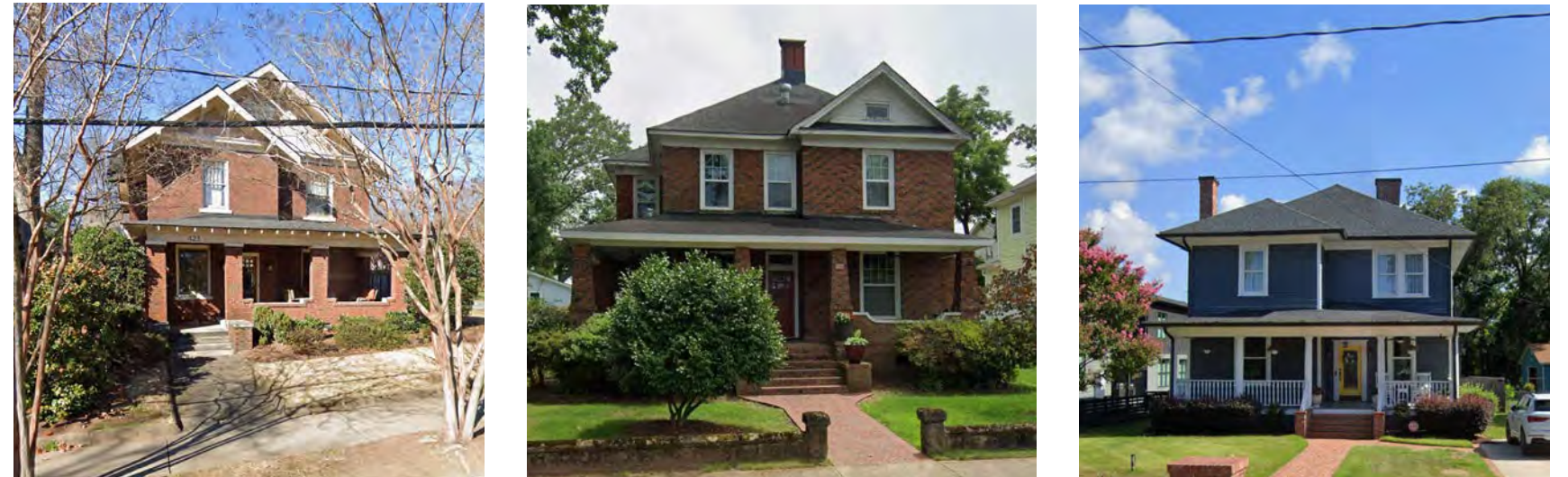
As shown here, all precedents found with an asymmetrical front gable have a hip roof porch (without further gables on the porch itself)
