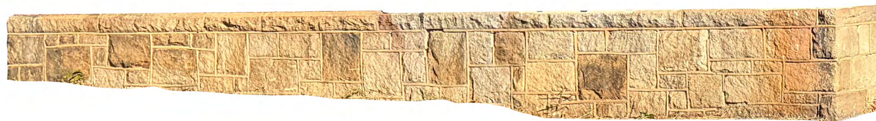
Granite Foundation Along 'back' western facade (to be re-purposed).
