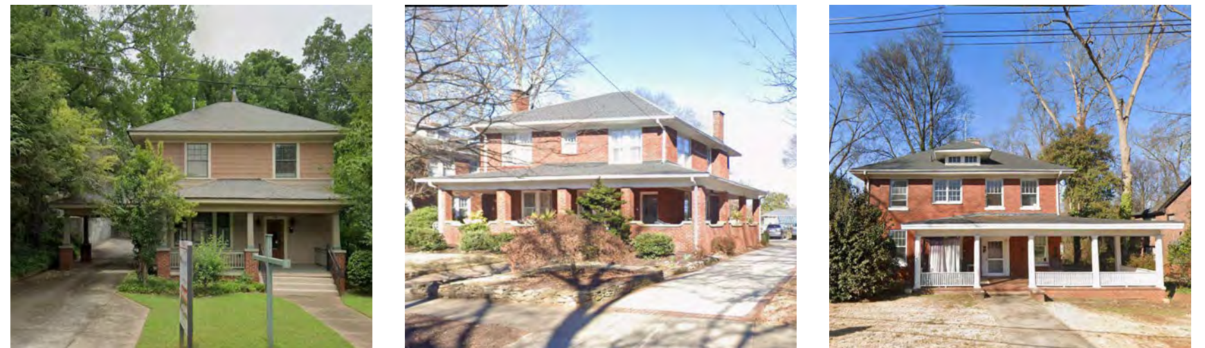
Many examples found feature a hip roof porch that is asymmetrical relative to the main house, often with an open corner.
