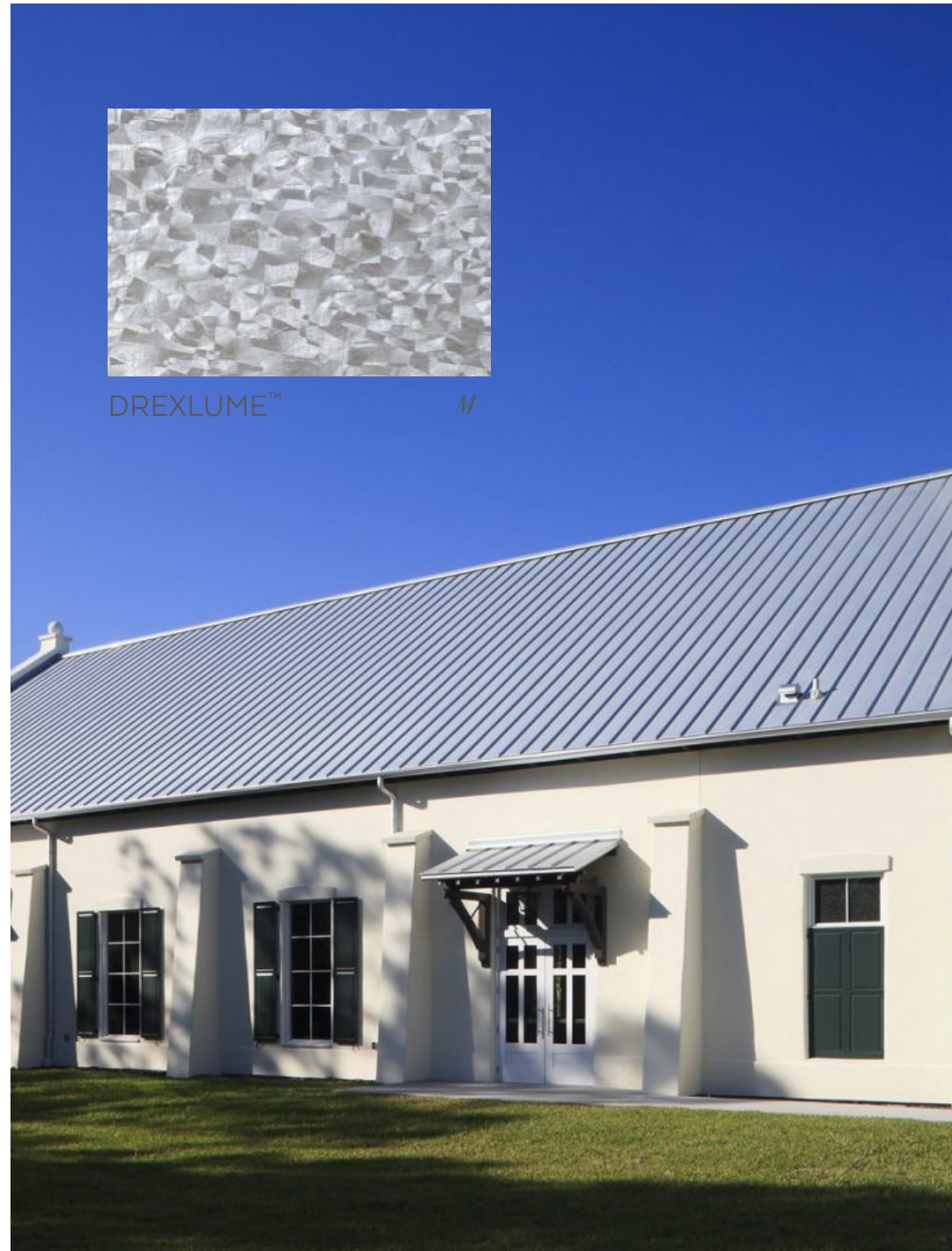
Reference roof from Jet Metals
