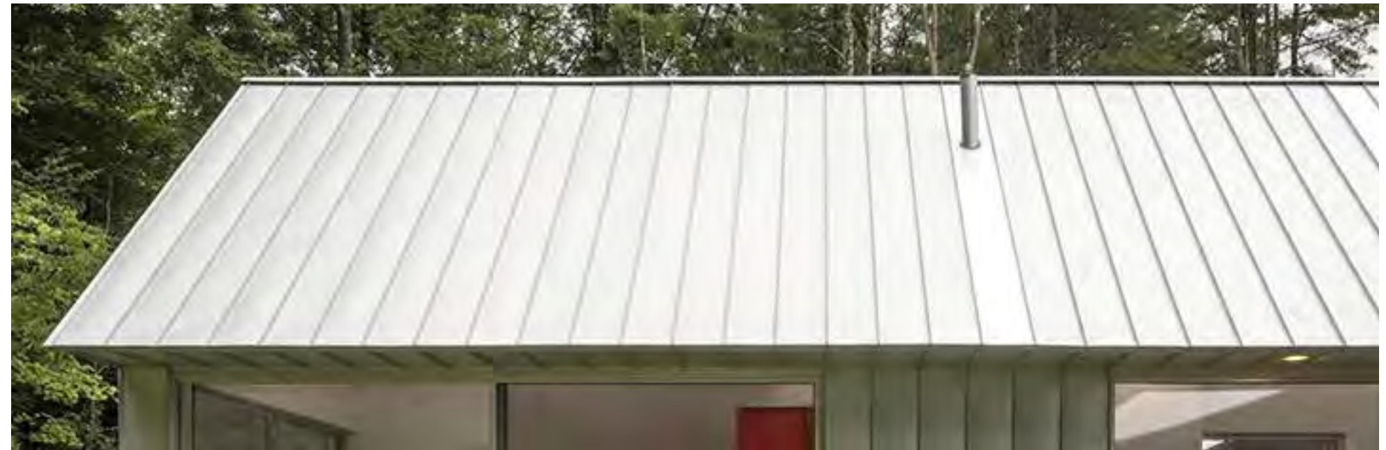
Reference image: The metallic roof will be highly active in the changing daylight and will help reflect solar heat gain.
