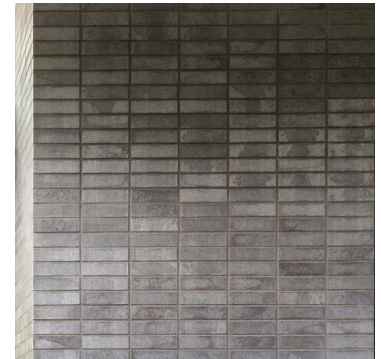
The brick will be used in a smooth stacked bond.
