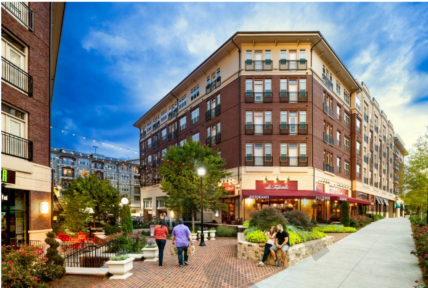
Generous sidewalks are constructed of durable and variable materials to highlight pedestrian pathways.
