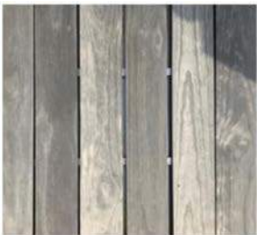
As Installed - Day 1
