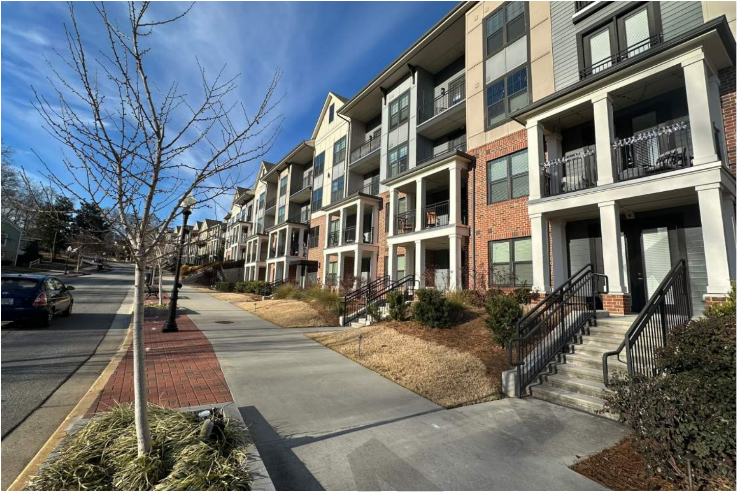
Residential entrances face the public realm with stoops that adjust for slope.
