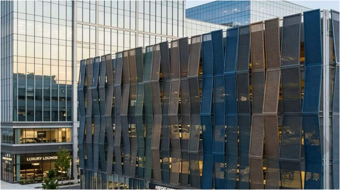
This garage is screened with a three-dimensional panels that limit the visibility of cars and interior lighting from the public realm.
