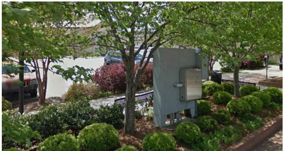
Utility box is located out of the pedestrian path in the landscape zone.
