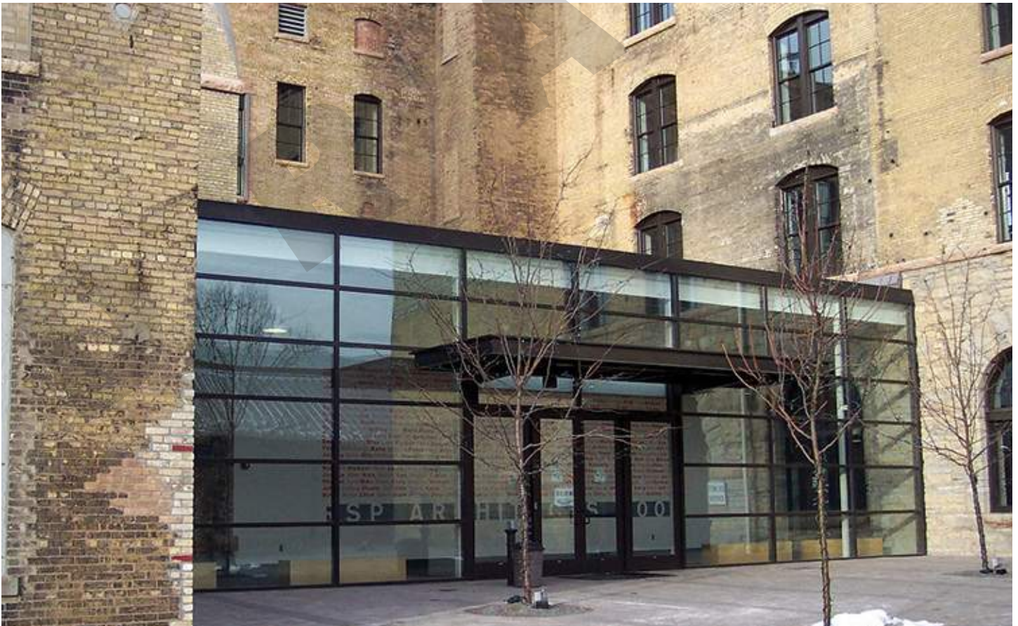
A glass connector distinguishes the new addition from the original structure while preserving existing architectural character.
