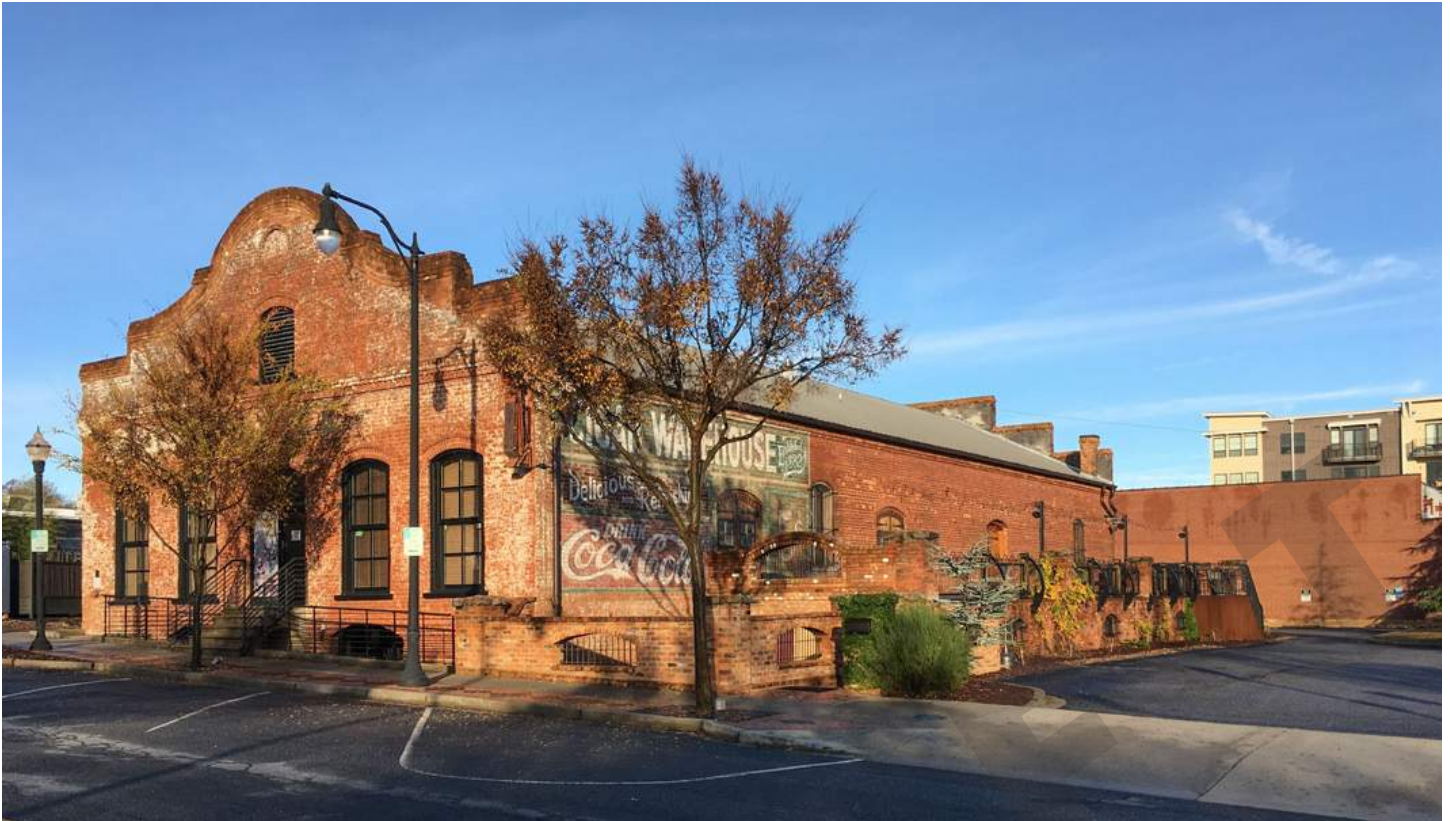
Adaptively reused masonry buildings retain their architectural character.
