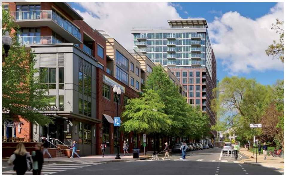
A stepped transition between a lower-scale brick building and a taller tower softens the height difference while maintaining a pedestrian-scaled street wall.
