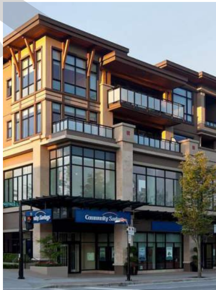
Recessed windows and cantilevered balconies add depth and rhythm to the upper stories.
